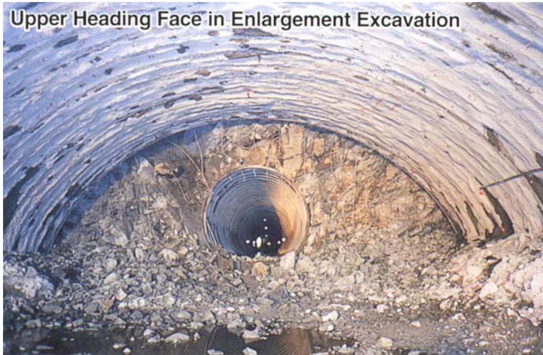
Figure 4.13: Pilot tunnel with pre-reinforcement and primary support of shotcrete and H100 beams. Top heading with completed primary support up to the face (courtesy: Japan Tunnelling Association).
