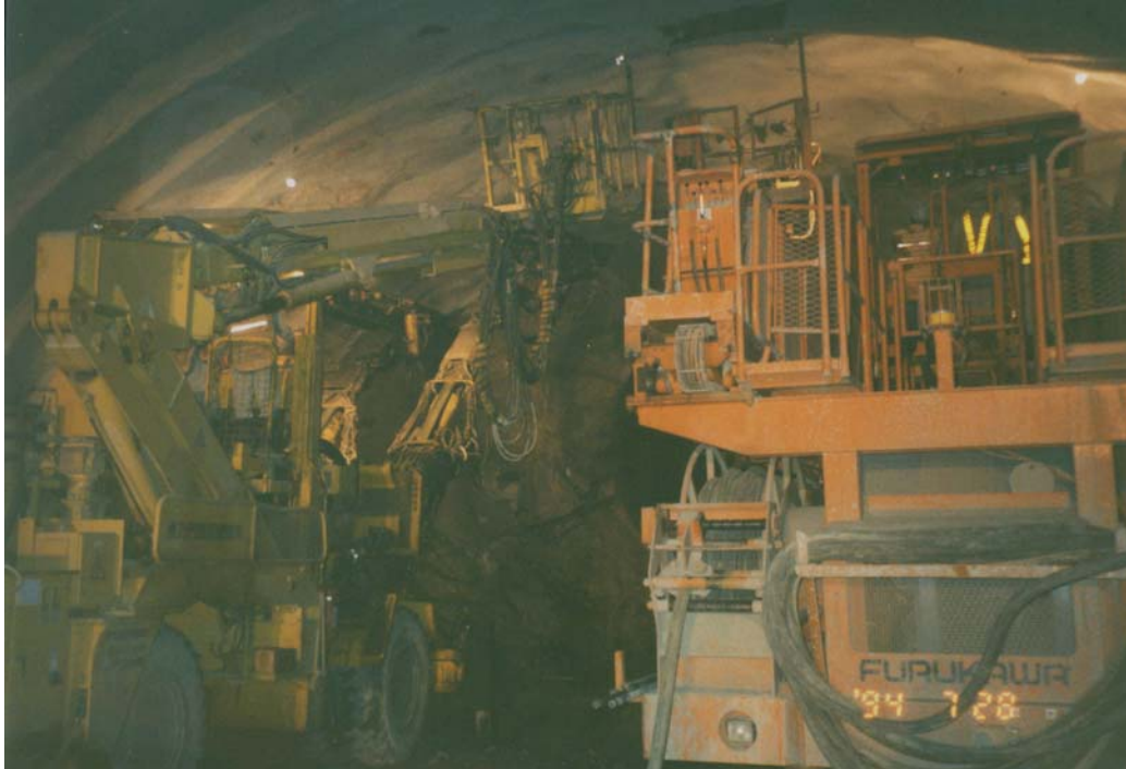
Figure 4.12: Drilling equipment used in Shimizu tunnel No.3.
