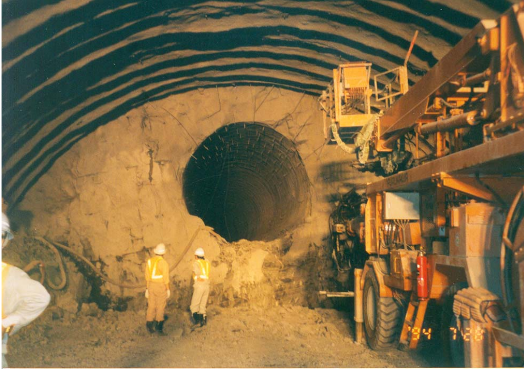
Figure 4.11: TBM pilot tunnel with pre-reinforcement and top heading excavation at Shimizu site. The destroyed plastic cables after blasting can be still seen. (note: illustrated dates are incorrect).
