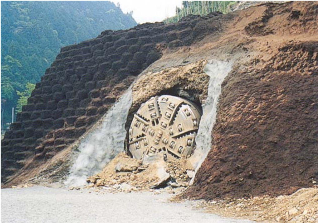
Figure 4.10 a,b: Breakthrough of the “Suruga” TBM.
