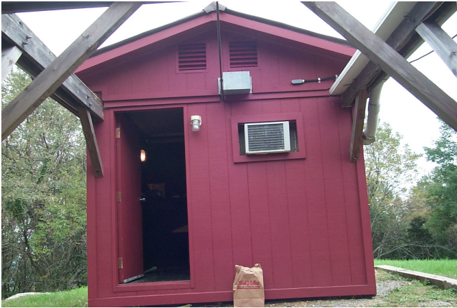
(a) View from under support structure.
