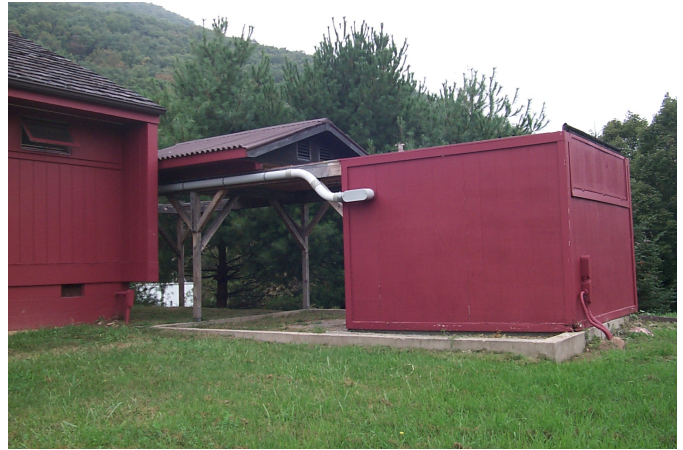
(b) View from west-southwest of building.
