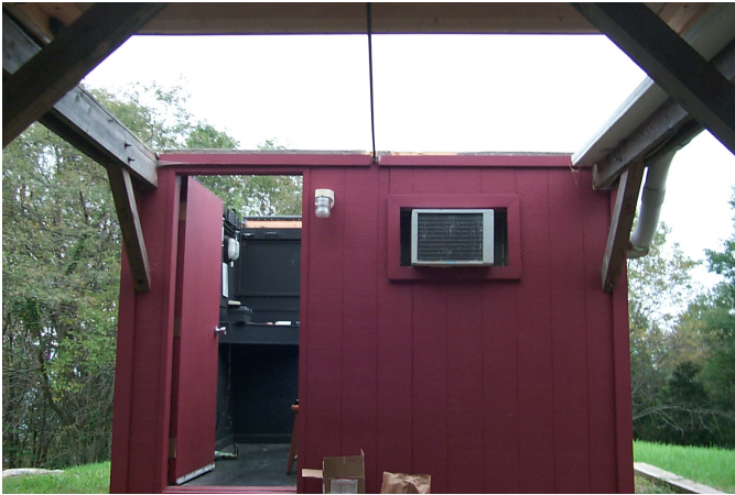
(a) View from under the support structure.
