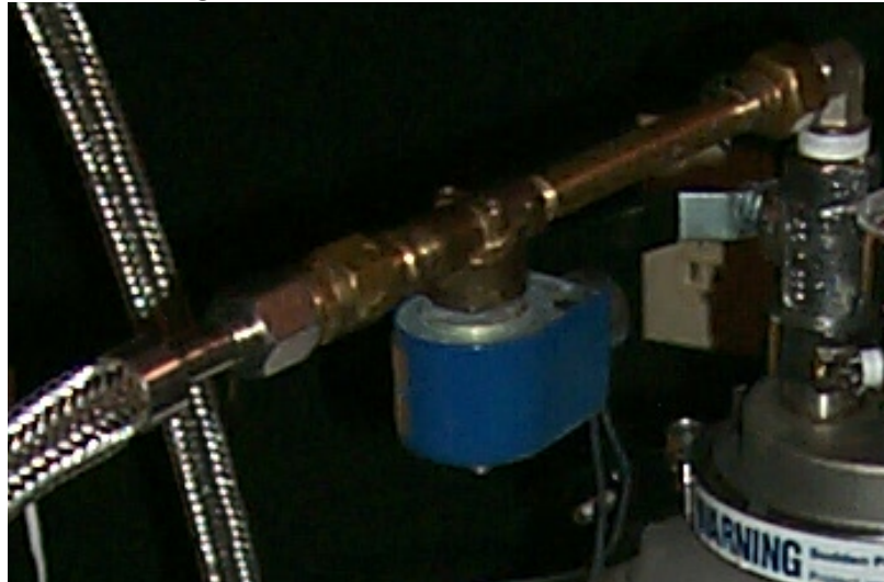
Figure 3.7: Close-up of the electric valve.
