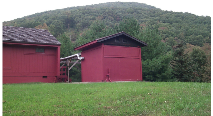
(b) View from southwest of building.
