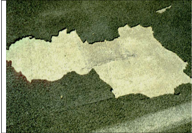
FIGURE 2. High-Friction Surface Raveling (Adam and Gansen 2001)
