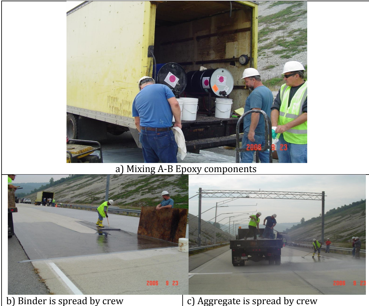
FIGURE 1. High-friction surface application (Adam and Gansen 2001).
