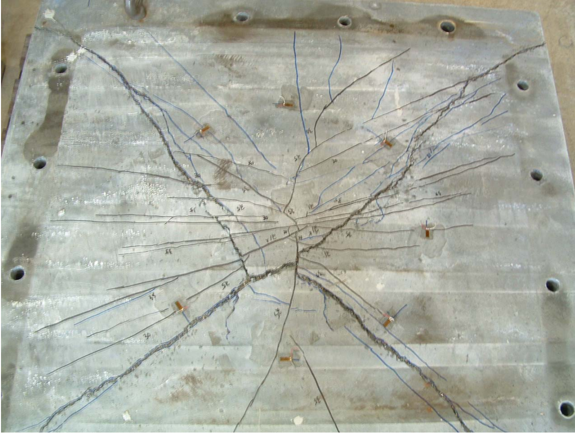
Figure B-48 – Failure Surface (3.0 in. slab – 2.5 in. plate)
