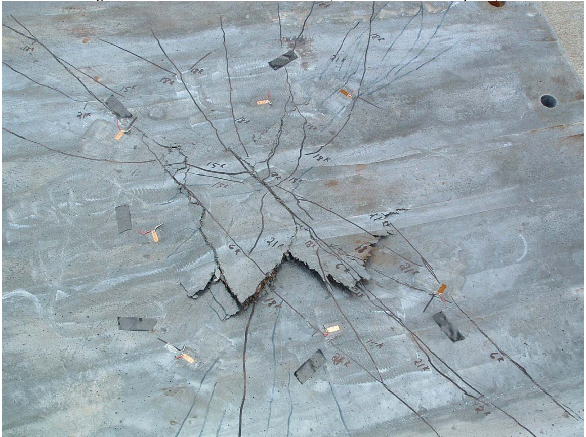
Figure B-18 - Failure Surface (2.0 in. slab - 2.0 in. plate)
