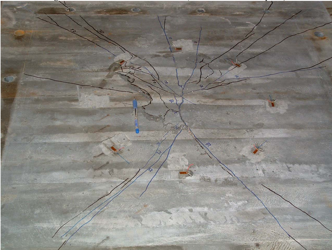
Figure B-53 – Failure Surface (3.0 in. slab – 1.5 in. plate)
