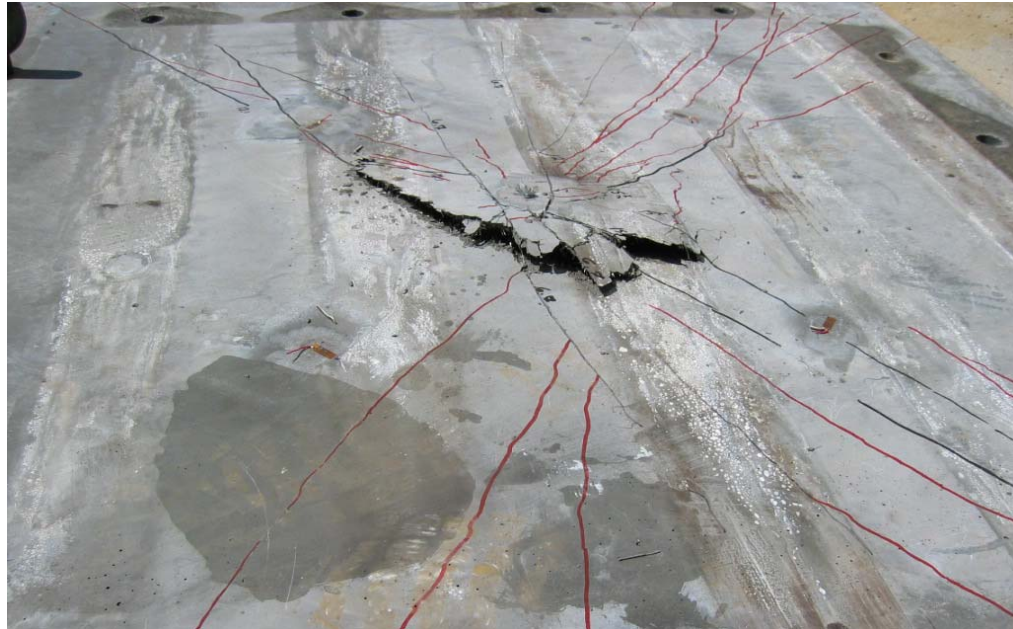
Figure B-13 – Failure Surface (2.0 in. slab - 1.5 in. plate)
