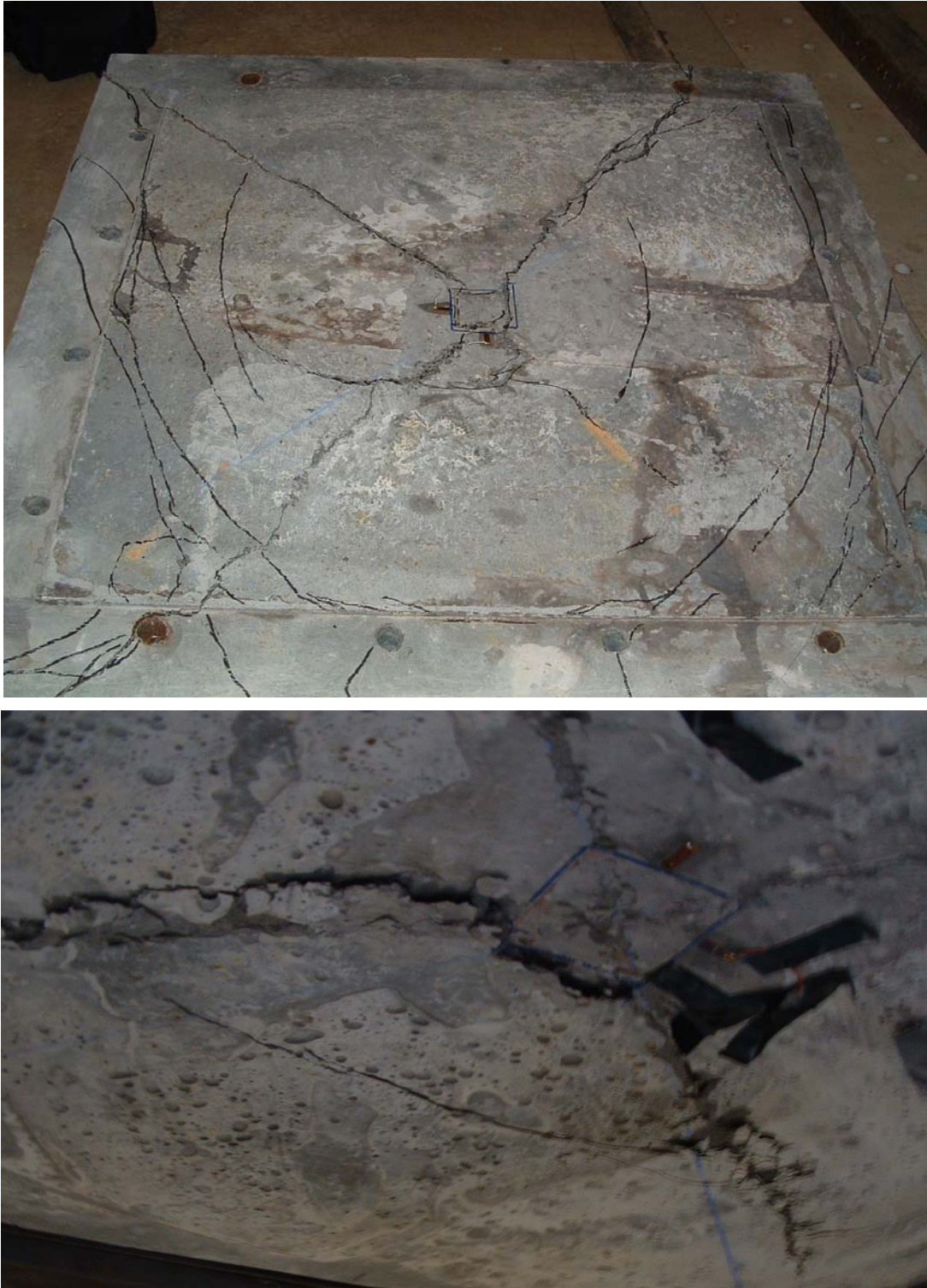
(b) Loading face of typical slab failing in flexure
