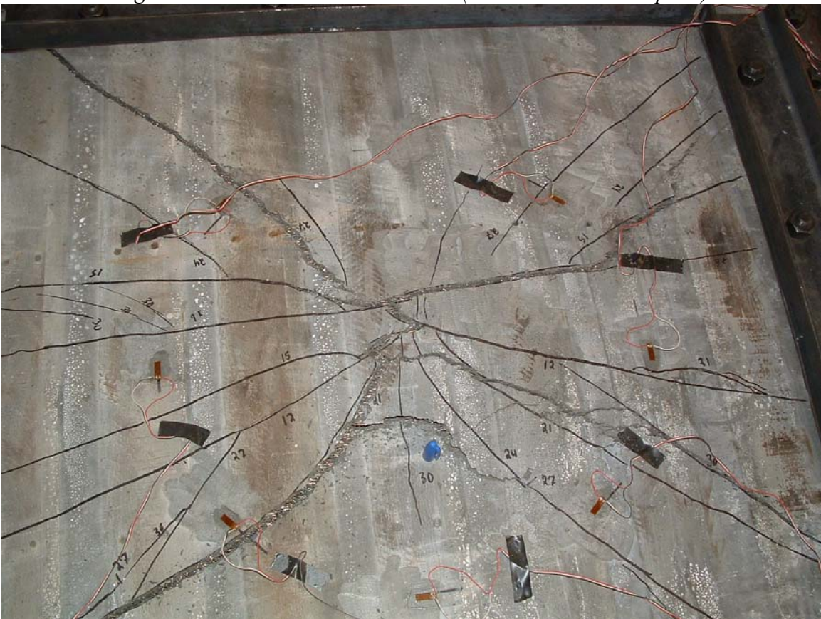
Figure B-43 – Failure Surface (2.5 in. slab – 2.5 in. plate)
