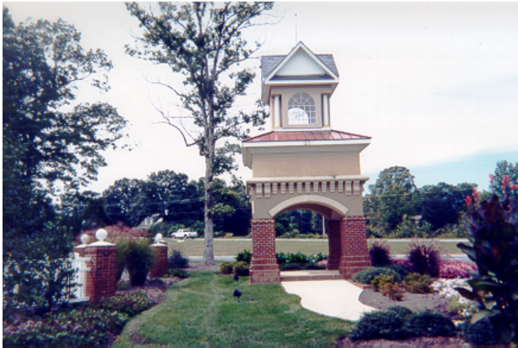
Figure 5 – Architectural Security Post Facade
