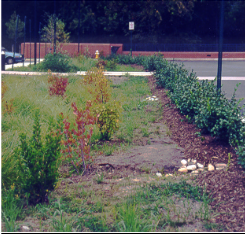
Figure 6 – Stormwater Management Barrier
