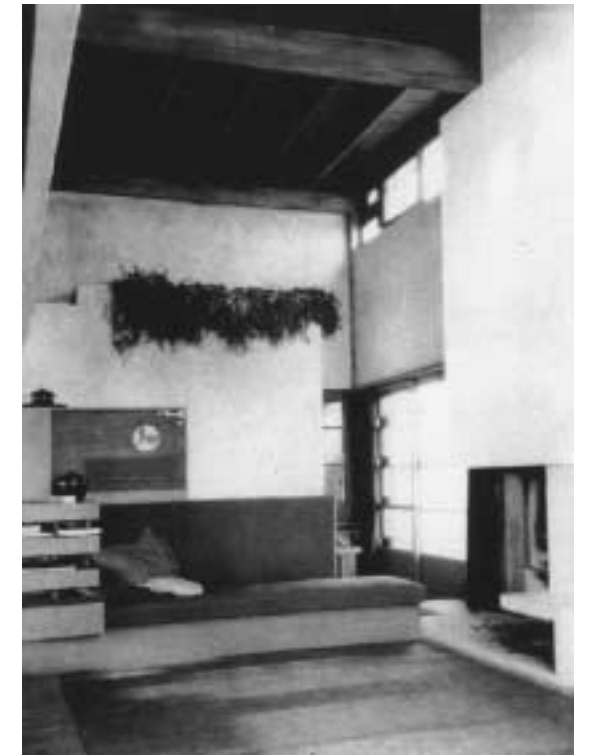
All furnishings, and fixtures for the Lovell Beach House were designed by Schindler. Each piece was built from the form-work used to fabricate the concrete frames.
