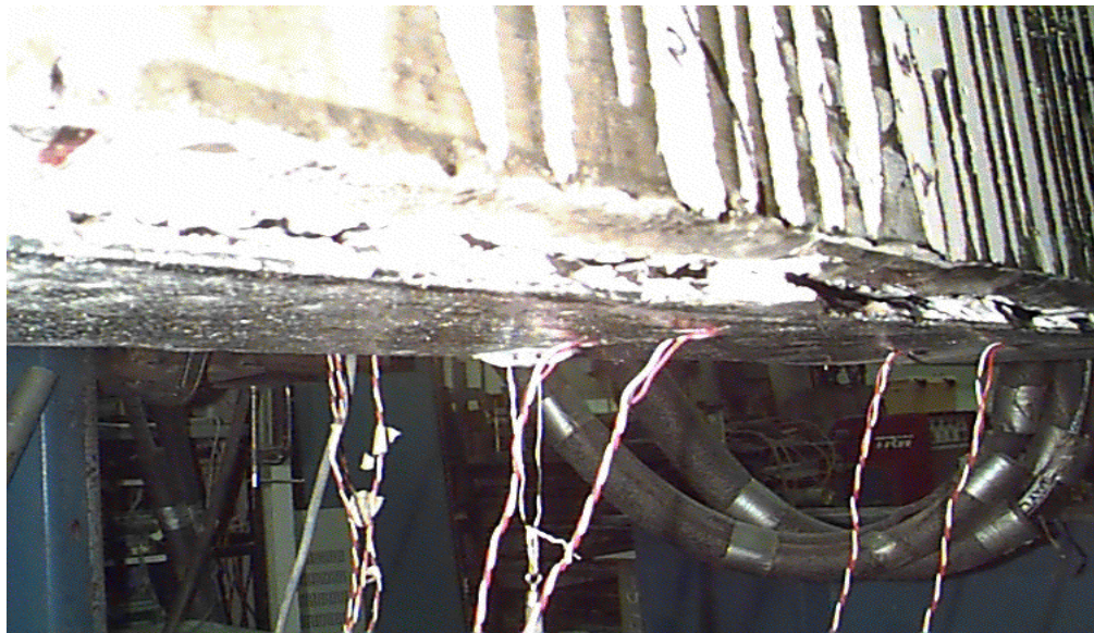
Figure 5.14: Debonding of the CFRP
