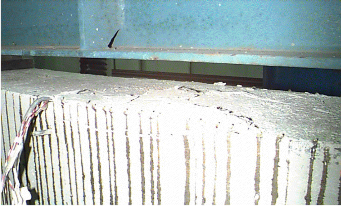
Figure 5.2: Crushing of the Concrete
