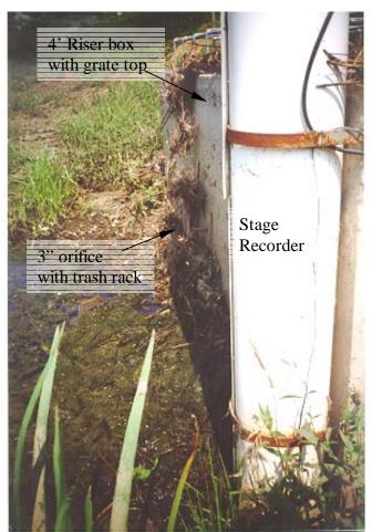
Figure 3-11. Oulet Structure After a Storm Event
