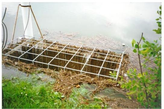
Figure 3-9. Top of Riser Box During an Overflow Storm Event
