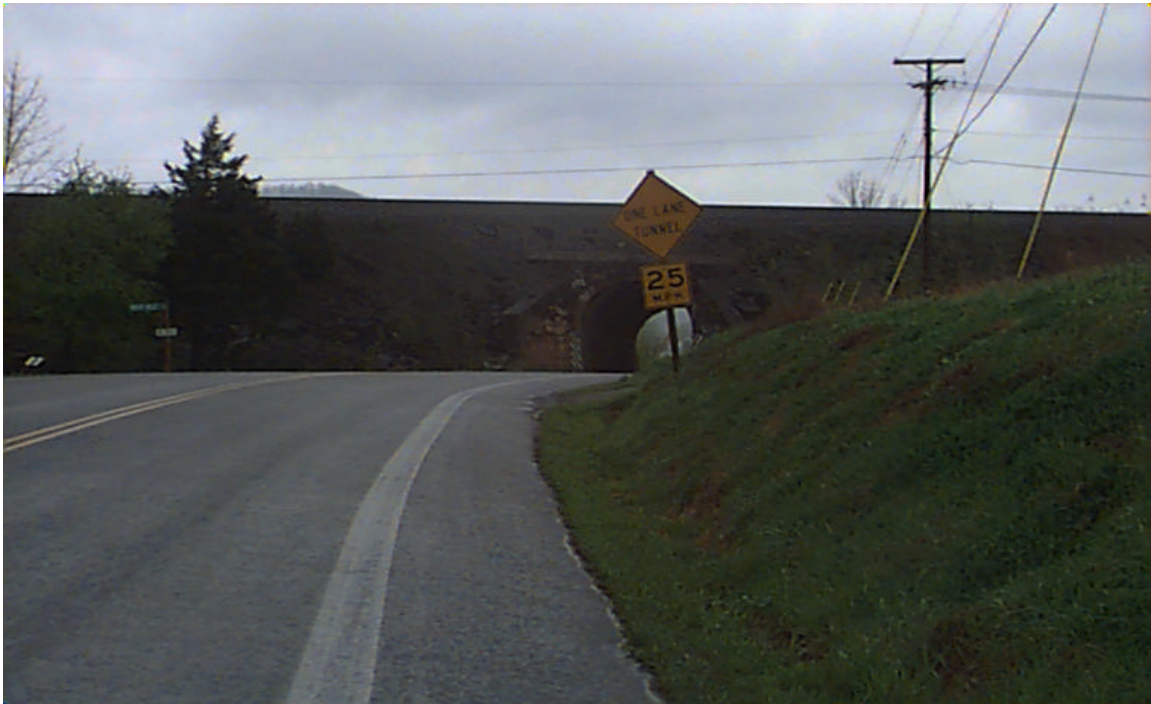
Figure A-4. Event 7: Marked One Lane Tunnel
