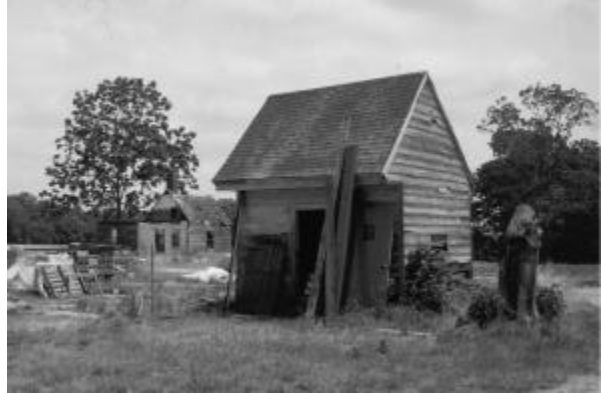
Figure 2.4 Looking northeast towards the dairy and the schoolhouse in the background. Author. June 1997.
