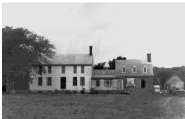
Figure 2.3 South side of Woodlands. Author. January 1997.
