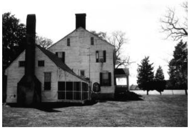
Figure 4.33 East side of Woodlands. Department of Historic Resources, Richmond, Virginia. 1966.
