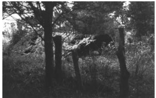
Figure 4.60 Wood shingled roof of a small outbuilding associated with the house near the wharf. Frank Strassler. November 1997.
