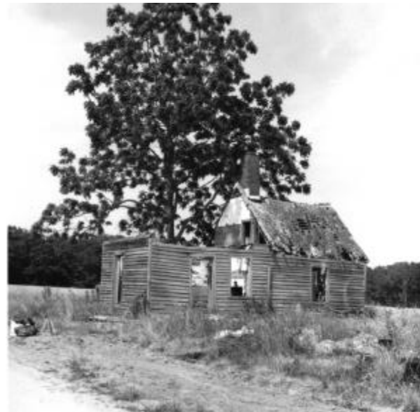
Figure 4.42 The schoolhouse, looking northeast. Since this photograph was taken, the wood structure of the building has collapsed with only the chimney standing. Author. June 1997.
