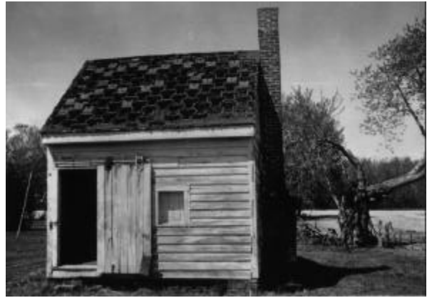
Figure 4.39 South face of outbuilding referred to as weaving shed. Department of Historic Resources, Richmond, Virginia. 1966.
