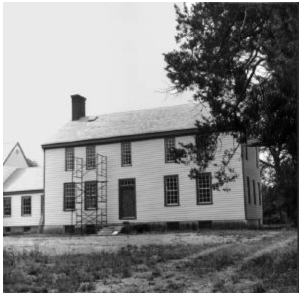
Figure 4.32 Woodlands with new colonnade-kitchen addition. Author. June 1997.
