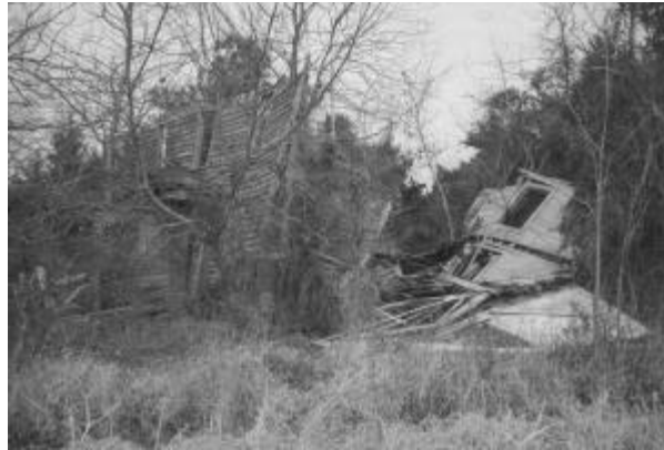
Figure 4.51 Decaying twentieth century farmhouse at Thomas's Wharf. Author. March 1997.
