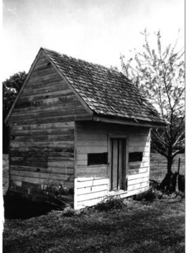
Figure 4.37 The dairy. Department of Historic Resources, Richmond, Virginia. 1966.
