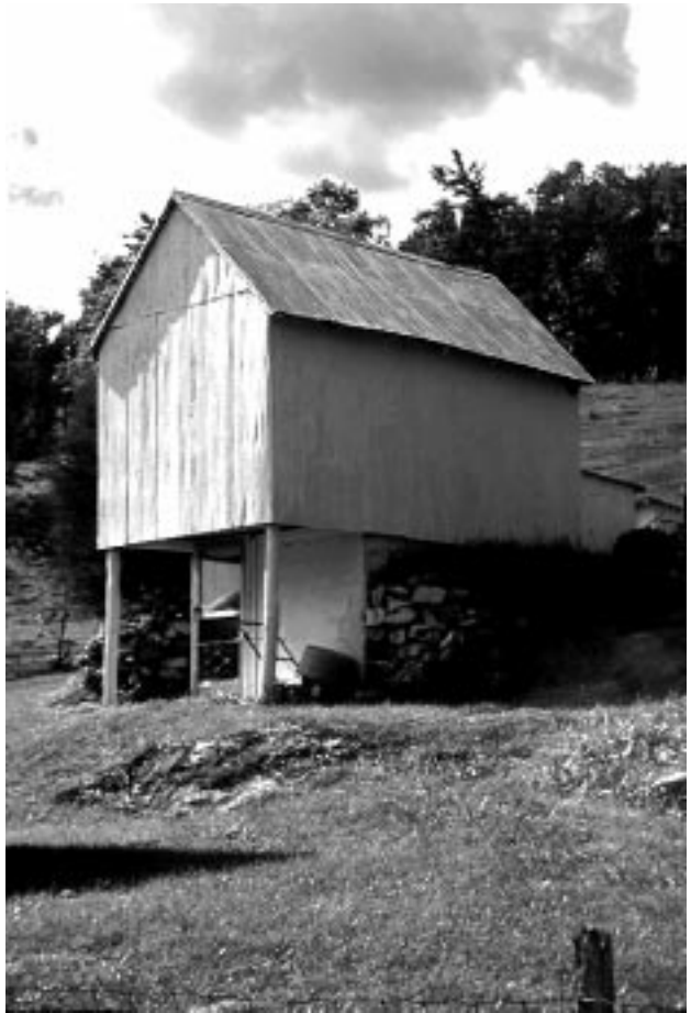
storage shed Montgomery County, Virginia
