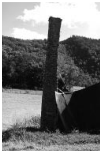
collapsed house Montgomery County, Virginia
