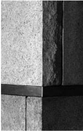
Carlo Scarpa column detail, Olivetti showroom Piazza San Marco, Venice, Italy
