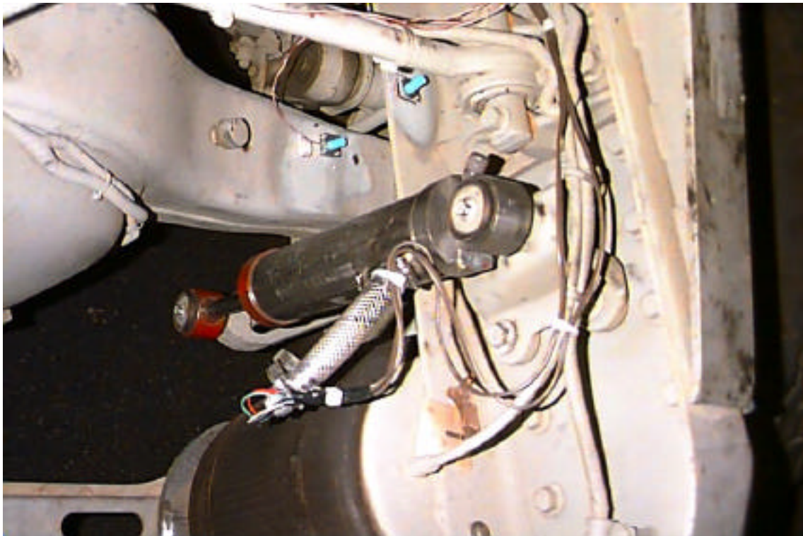
Figure 5.1. Installed Semiactive Damper and Accelerometers.
