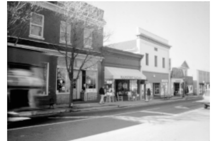
41 Main Street Facades
