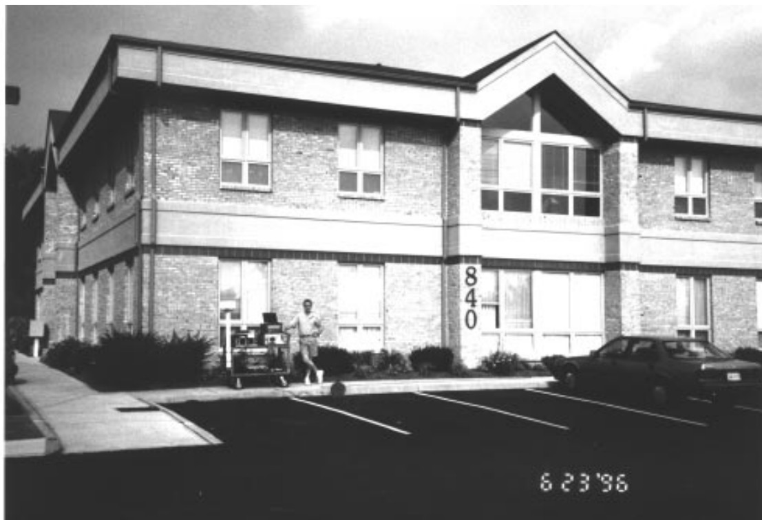
Figure 5.8: Photograph of the receiver at Site 2 measurement location Rx12
