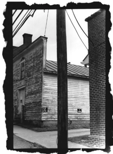
The presence of telephone poles and unpainted facades impact the streetscape.
