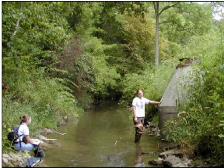
Service-learners take note of an exposed pipe (a sewer manhole) located on the banks of Stroubles Creek
