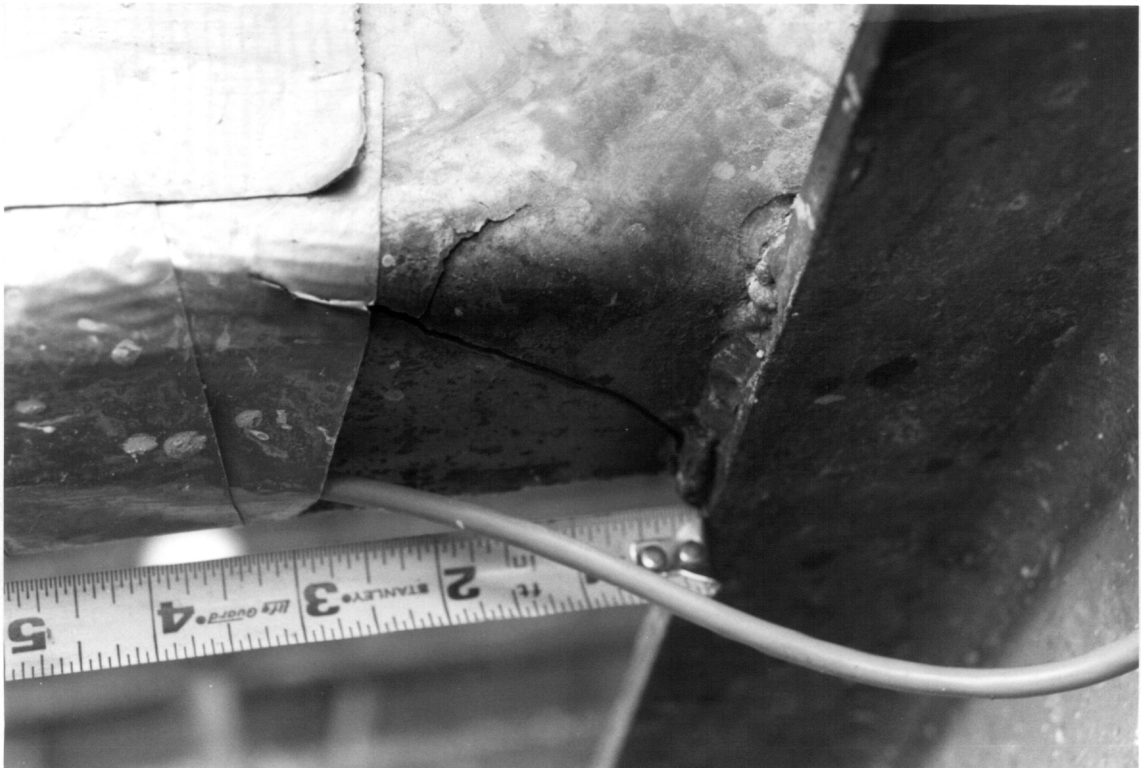
Figure 121. The Crack Propagated around the Bolster Leaving Reduced Effective Cross-Section; The bolster failed by plastic deformation a week after this photo had been taken.
