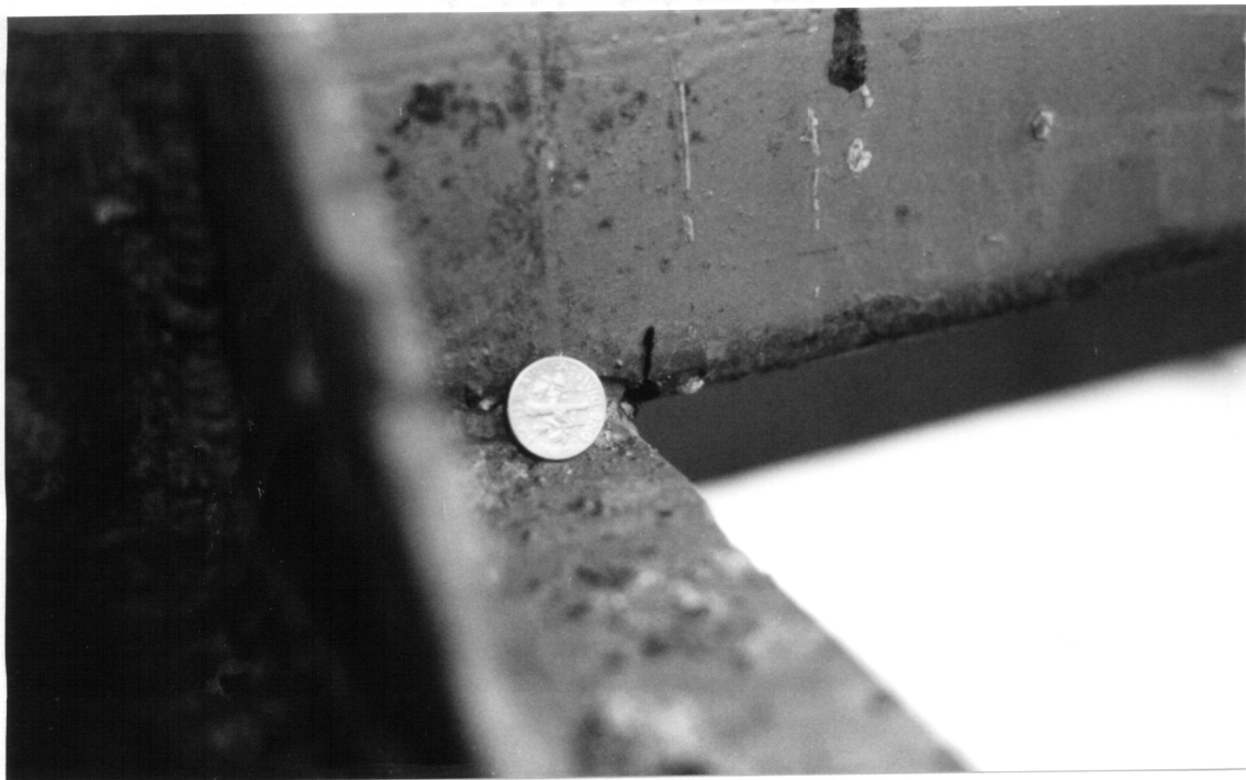
Figure 116. Fatigue Crack in the Inside Section of the 3rd Bolster of the Full-Tree Trailer.
