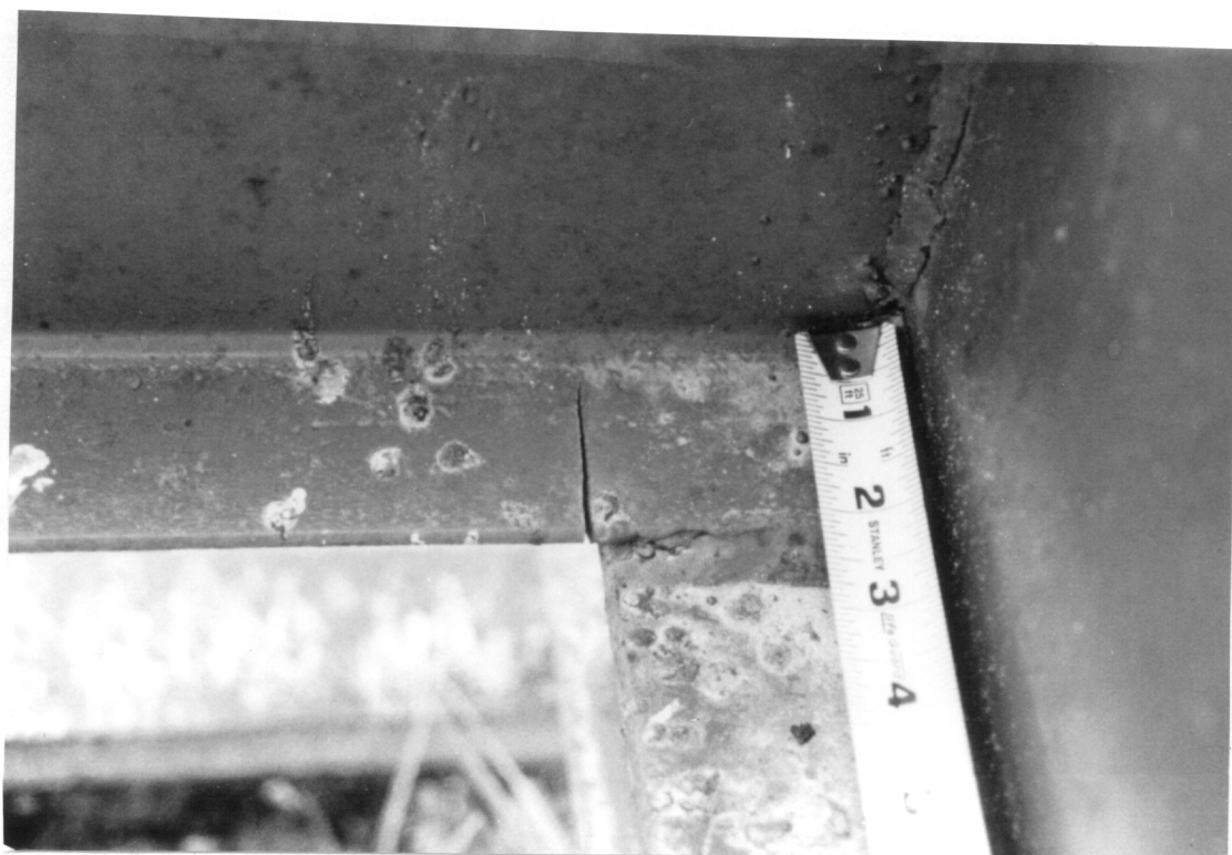
Figure 117. Fatigue Crack at the Corner Where the Flange of the Cross Member is Welded to the Flange of the Main Beam.
