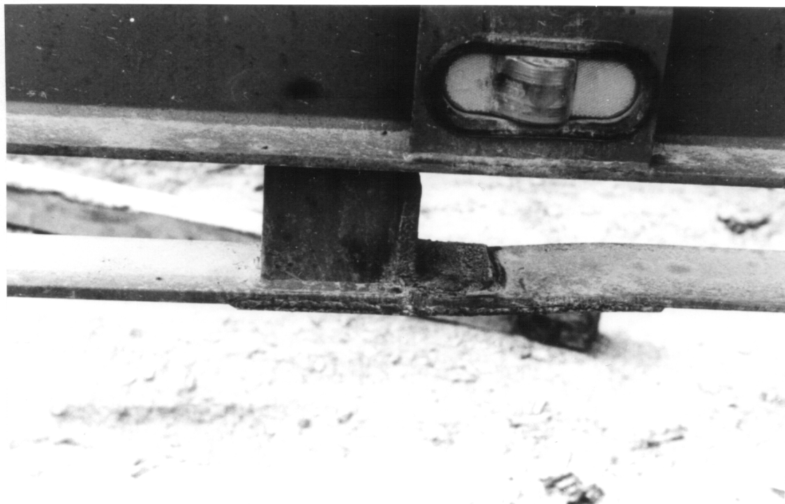
Figure 118. Fatigue Crack in the Bow-String Truss under Main Beam.
