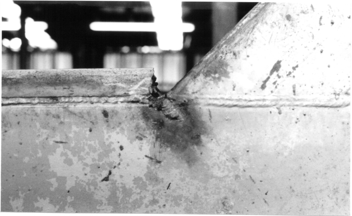
Figure 112. Fatigue Crack Inside of Standard and Bolster Junction.
