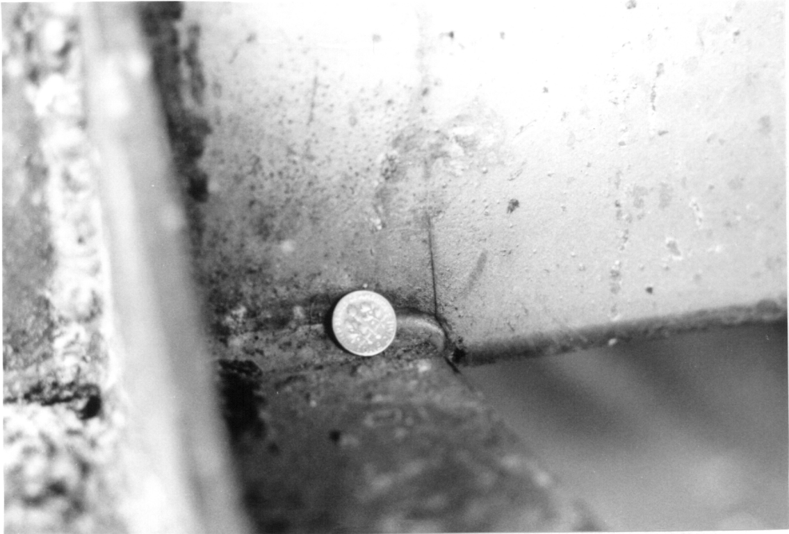
Figure 115. Fatigue Crack in the Outside Section of the 3rd Bolster of the Full-Tree Trailer.
