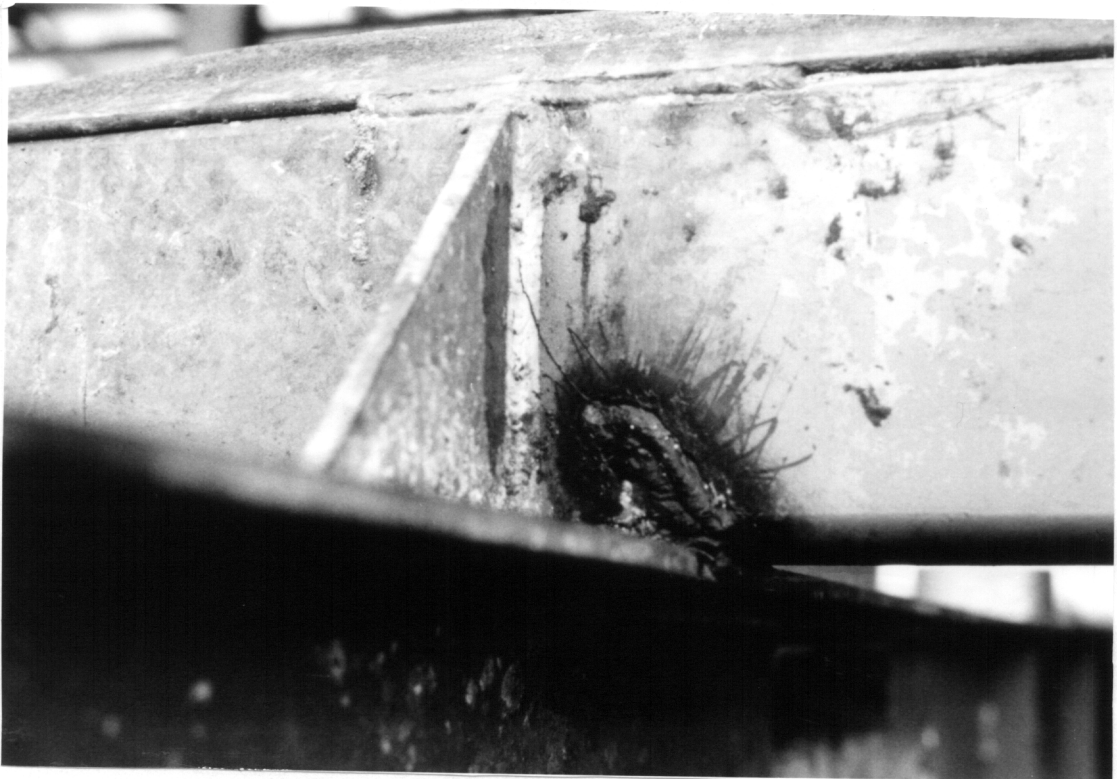
Figure 113. Fatigue Crack at Bolster and Main Beam Weldment.
