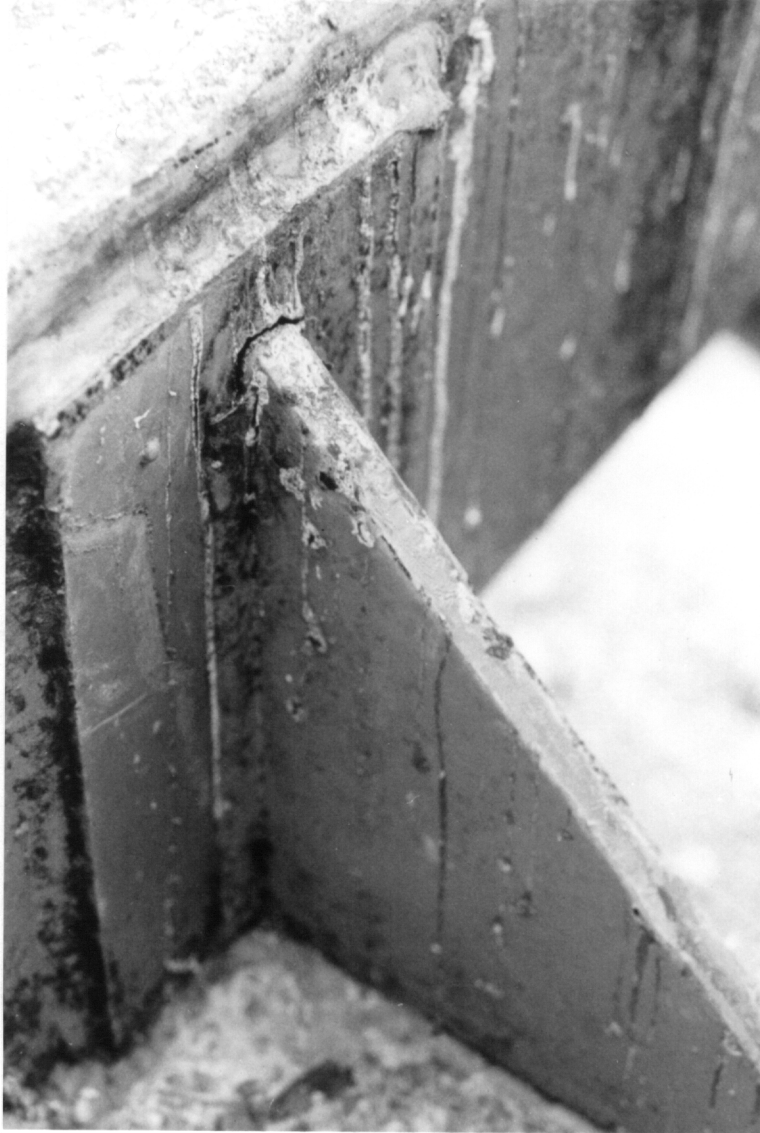
Figure 114. Fatigue Crack at the Tip of the Bolster Reinforcing Gusset.
