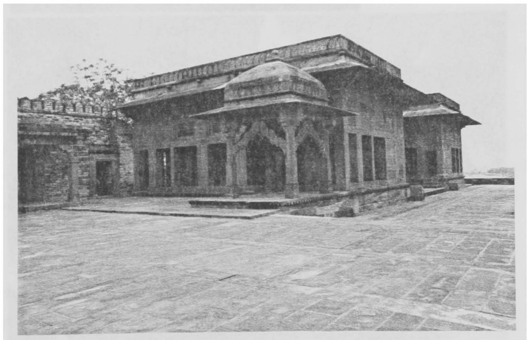
Figure 6-40: The treasury (Fatehpur Sikri) The eave at the roof level projects around the building. This projected portion provides a line of continuity to the structure.
