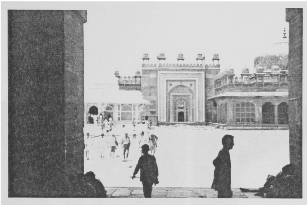
Figure 6-113: Dummy gate in the north wall (Fatehpur Sikri)
