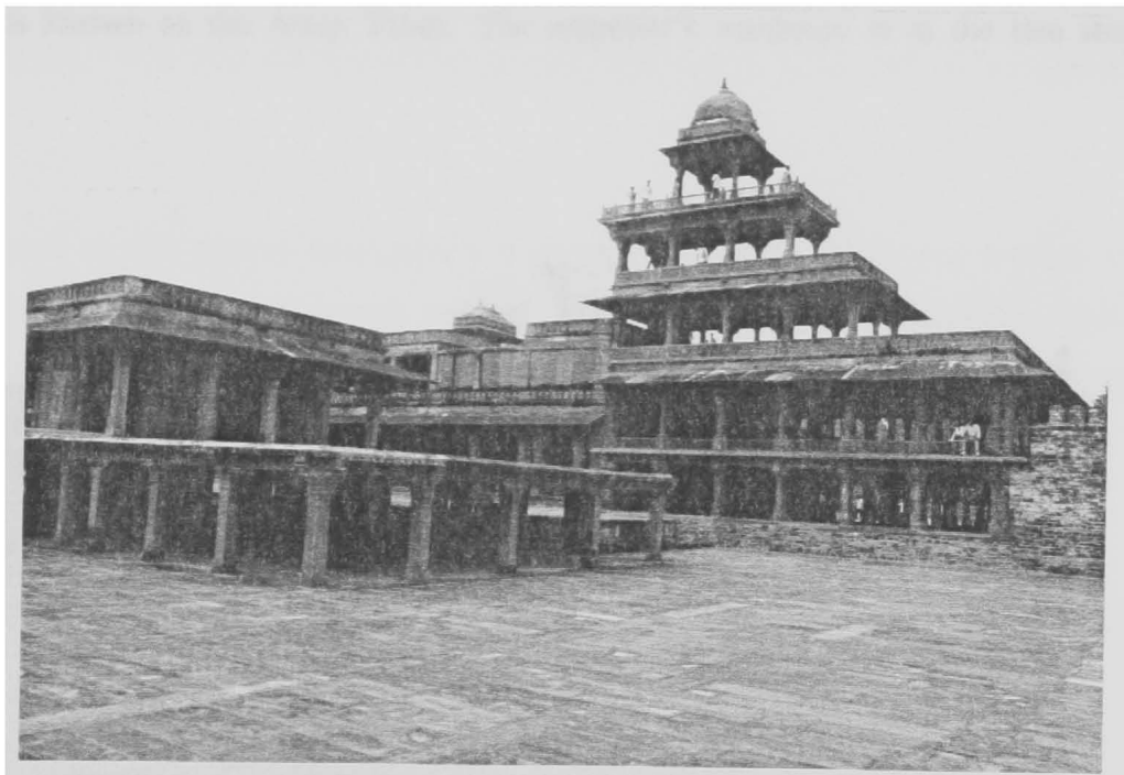
Figure 6-53: Madarasa (Fatehpur Sikri) This building is located east of the Panch Mahal. It may have served as the Madarasa or school for harem children. It follows the architectural form and style of the other buildings.
