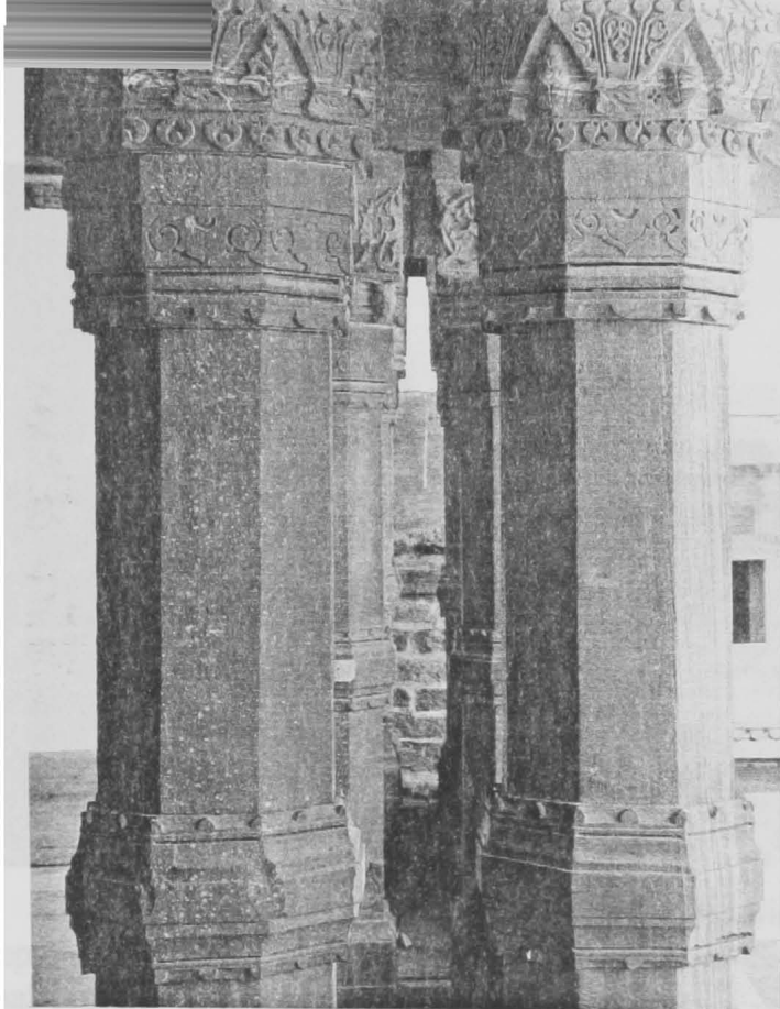
Figure 6-48: Panch Mahal (Fatehpur Sikri): column details
