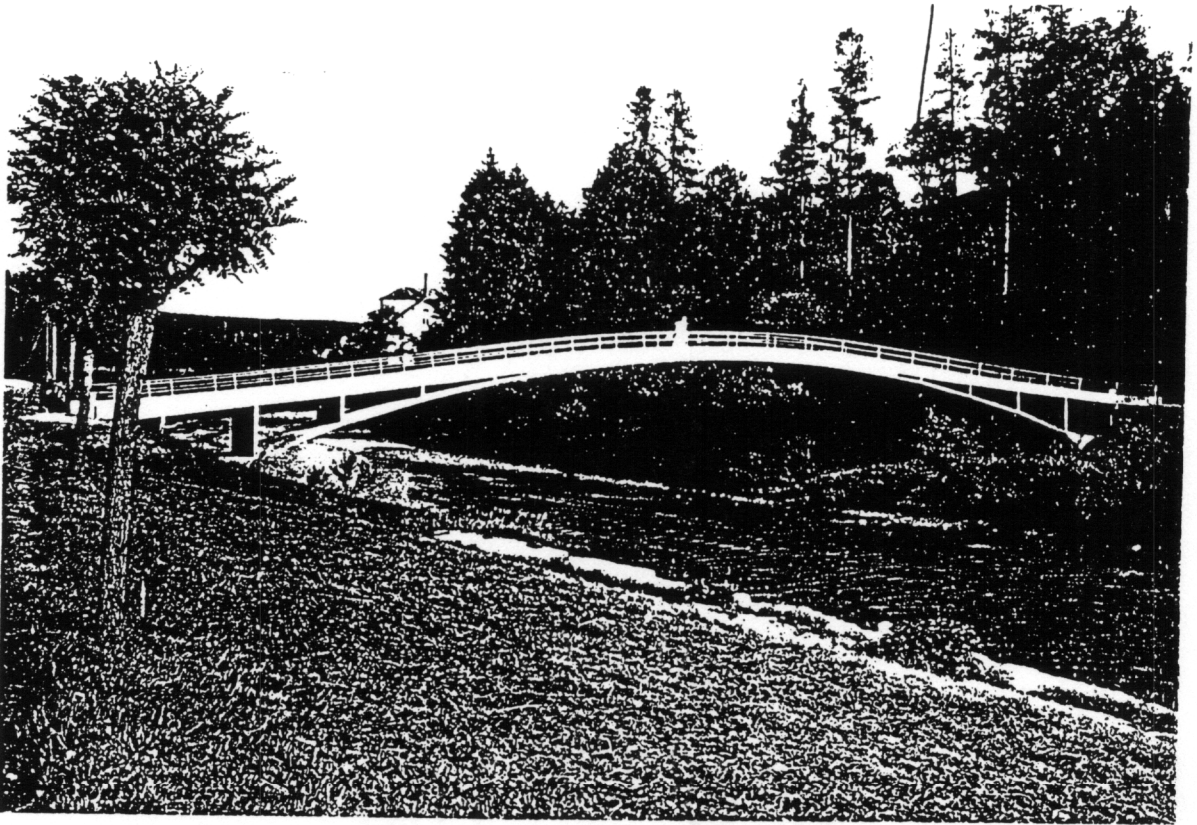
Figure 103. Bridge over the Toess near Wulflingdon, Switzerland. (Michaels, 1950, p. 80)
