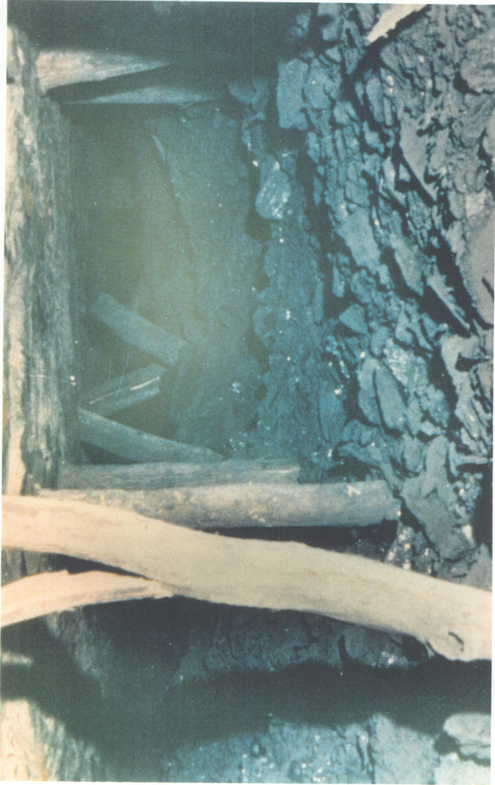
Figure A.18—Condition of crosscut between pillars E and F, location 1, fig. A.17, VP No. 3 Mine (After Campoli, et al., 1990a).
