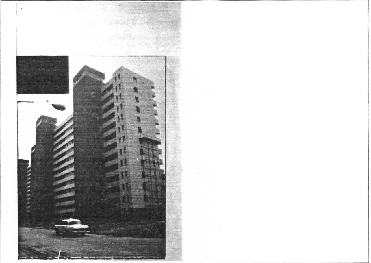
Figure 67. A High-rise apartment complex
