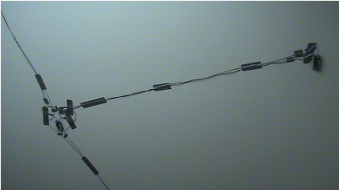
Figure A.4: A portion of the beacon network installed on the ceiling. All beacons were hard-wired to avoid complications with weakened batteries.
