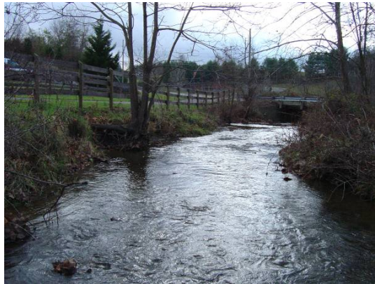
Figure 3.1. Bridge downstream of shrub reach cross-section.
