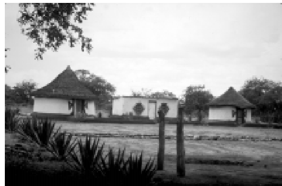
ground treatment - Venda, Dite Area
