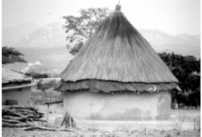
thatch over metal disc roofing roadside dwelling, Masvingo-Chimanmani road
