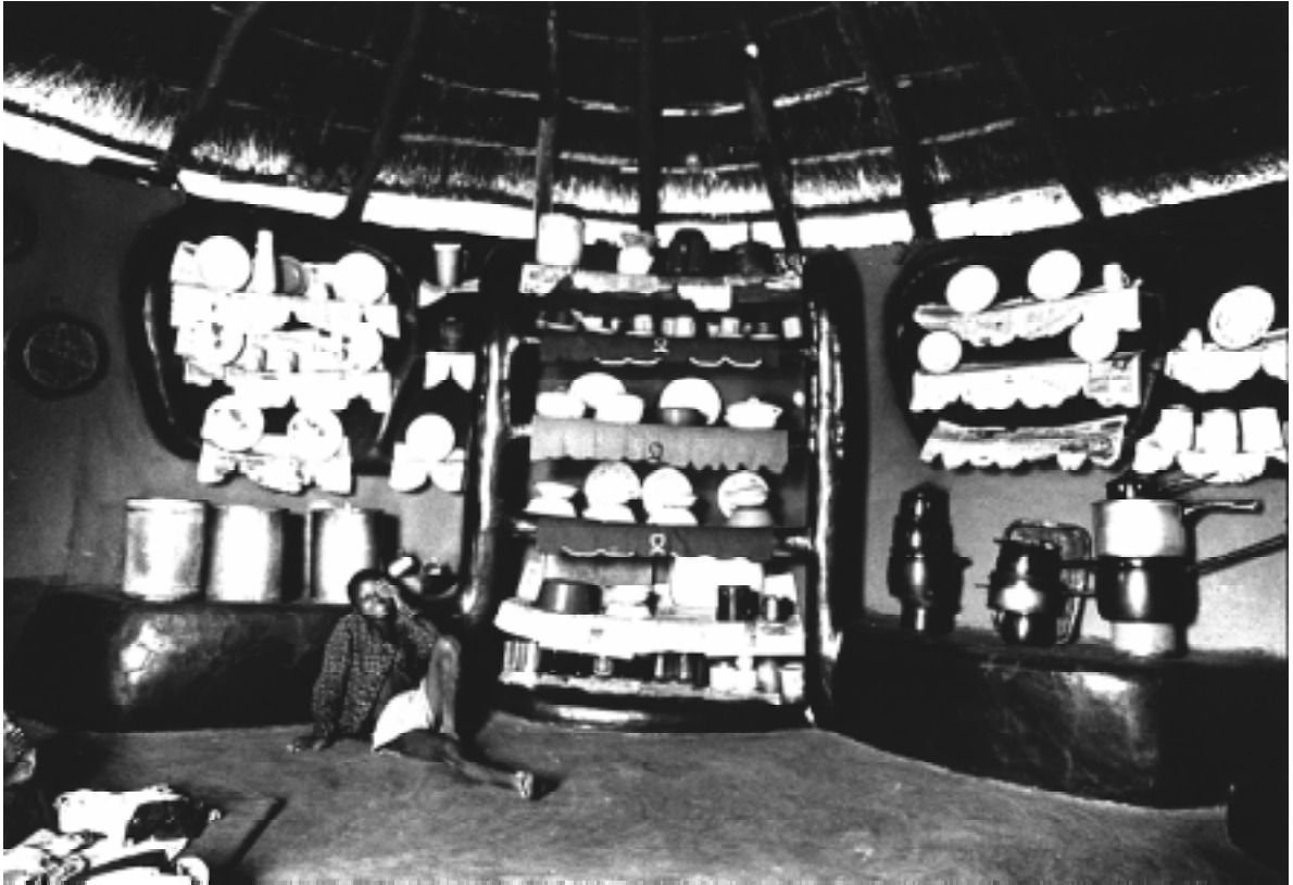
interior of kitchen hut; walls and storage are pounded earth, roof is thatch
