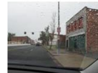
Figure 10. Intersection of H street and 3rd street
