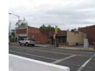
Figure 11. Two temporary buildings
