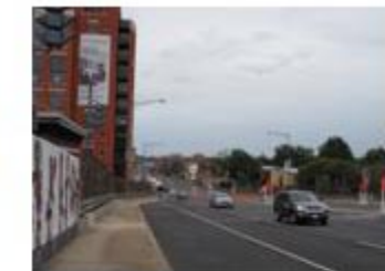
Figure 8. View from the west to the site
