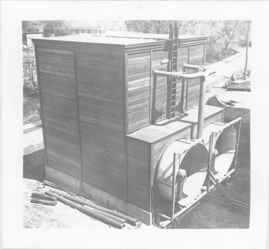
Fig. 11. The V. P. I. Cooling Tower with Test Equipment Installed
