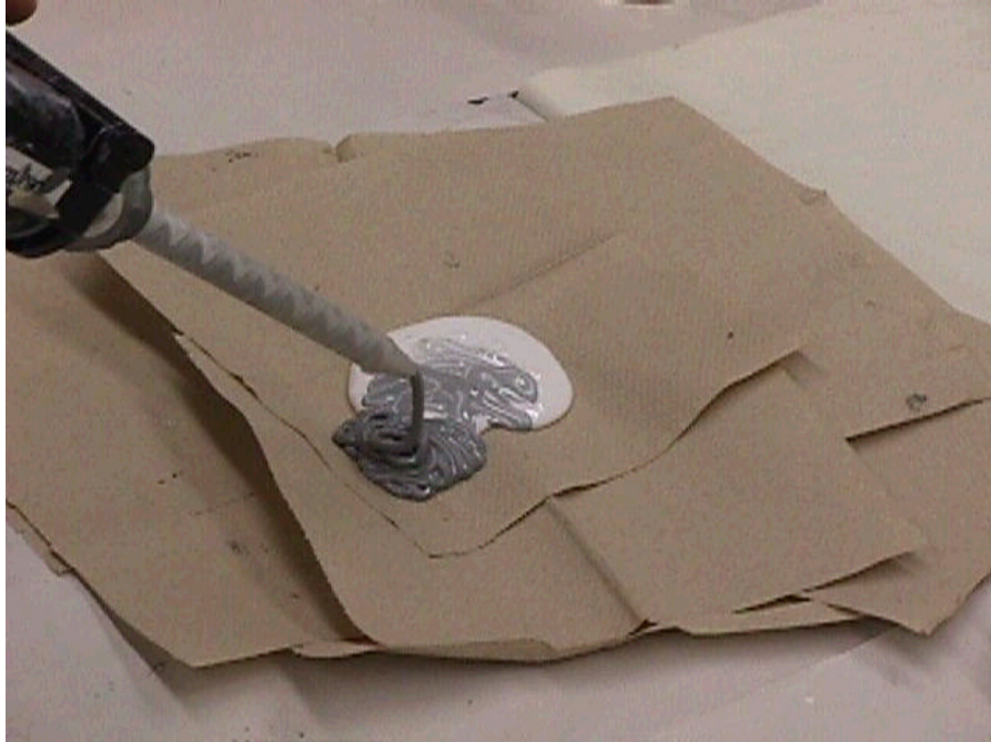
Figure A.11 Insuring that sealant components are mixed adequately before application
