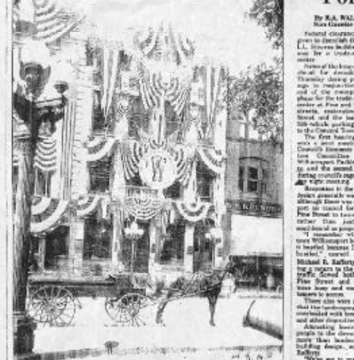
SOON TO BE DEMOLISHED is the former West Branch National Bank building, which became part of the L.L. Stearns and Sons department store after the bank moved to Pine and West Fourth streets in 1917...
