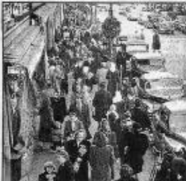
REPAIRS MADE, DOWNTOWN WAS BEEN Shoppers along Pine Street in 1940
