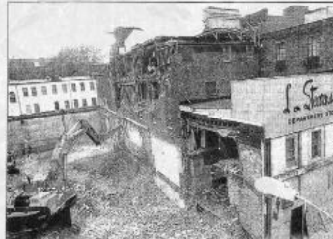
WIDEN WALLS CAME TUMBLED DOWN Heavy equipment pulls away the former L.L. Stearns & Sons building of West Third and Laurel streets...
