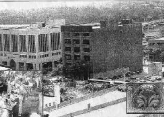
AS THE AGING BUILDING COMES DOWN, A MODERN LOOK BEGINS TO EMERGE An old home base atop the Stearns. Demolition is a large job of rubble...
