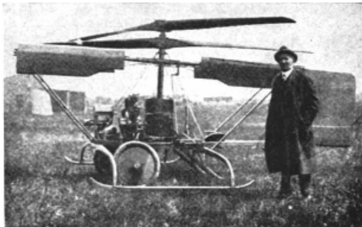
Figure 2.3: Berliner Coaxial Helicopter ( www.centennialofflight.gov )
