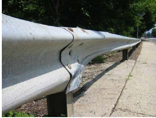
Figure 53. Minor Rail Deflection to a Strong Post W-Beam Barrier
