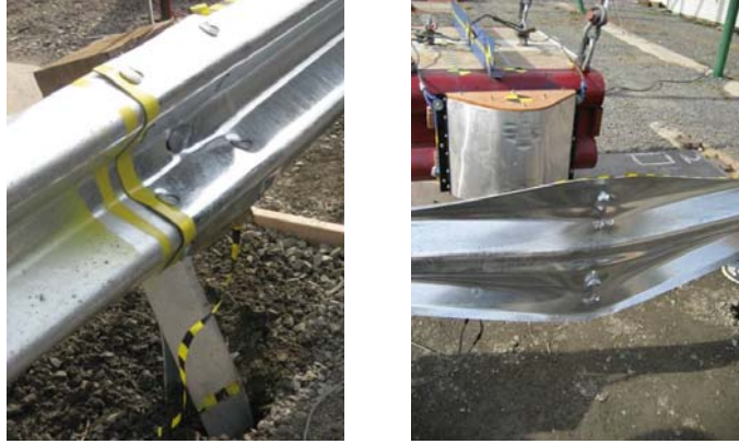
Figure 24. Splice Damage (left) and Impact Location Damage (right)
