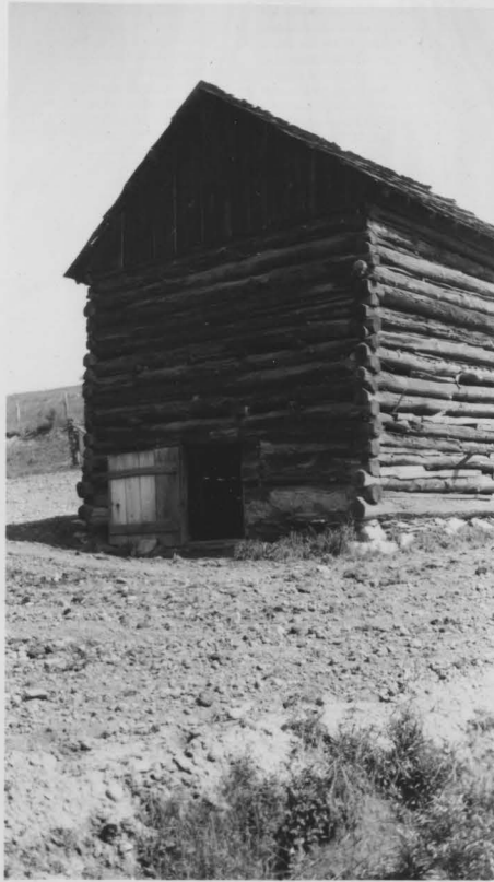
Figure 10. Abandoned Flue-Cured Tobacco barn. This barn is now used for storage.
