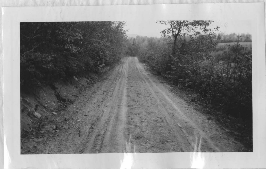
Figure 7. Dirt road in Land Classes I and II combined, area. This is a better than average road for the entire area. Excavation along this road reveals considerable mica in the formation.
