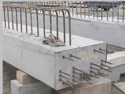
Concrete (compression) and metal (tension) working together in a beam
