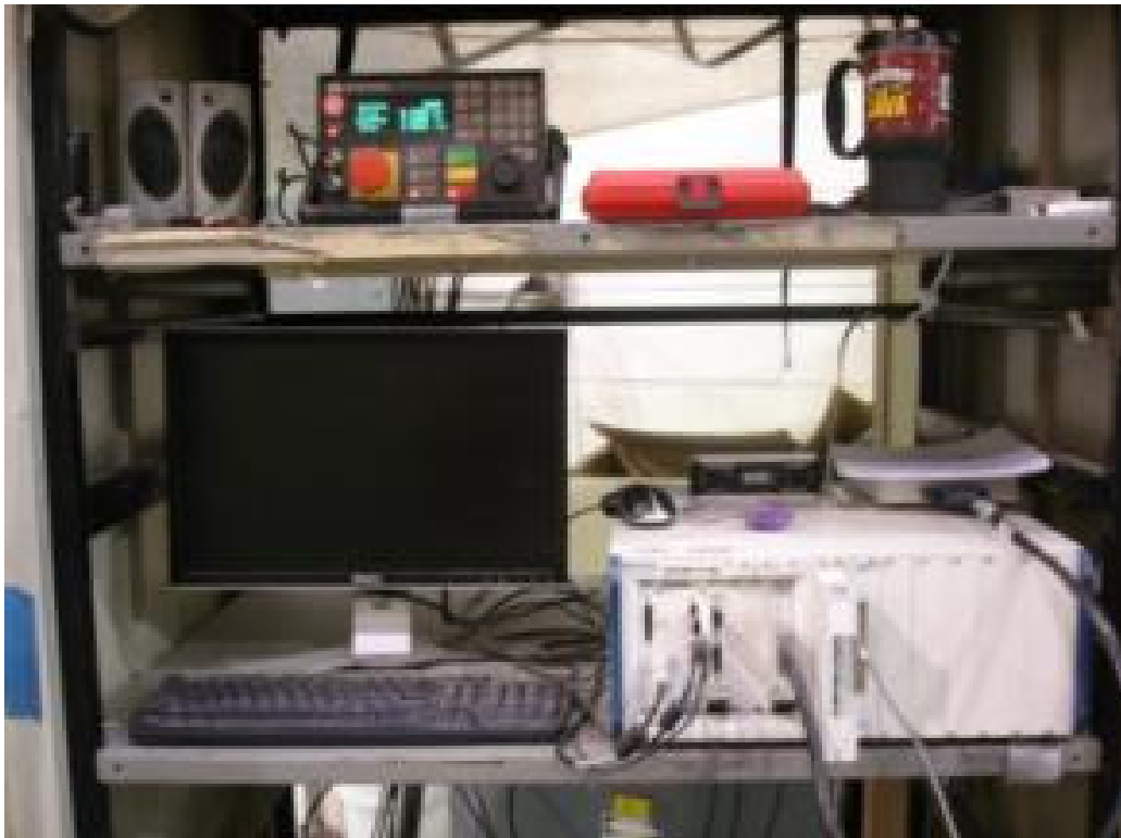
Figure 2.18. MTS 407 controller and NI data acquisition system
