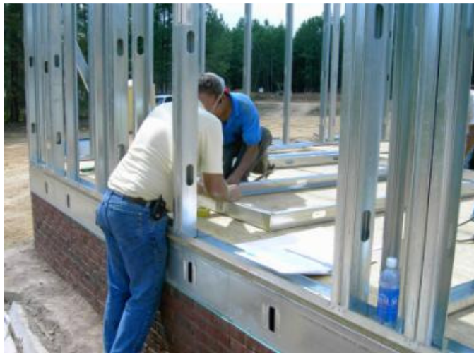
Figure 1.4. Web holes are provided in the supporting beams (photo courtesy of Steel framing)
