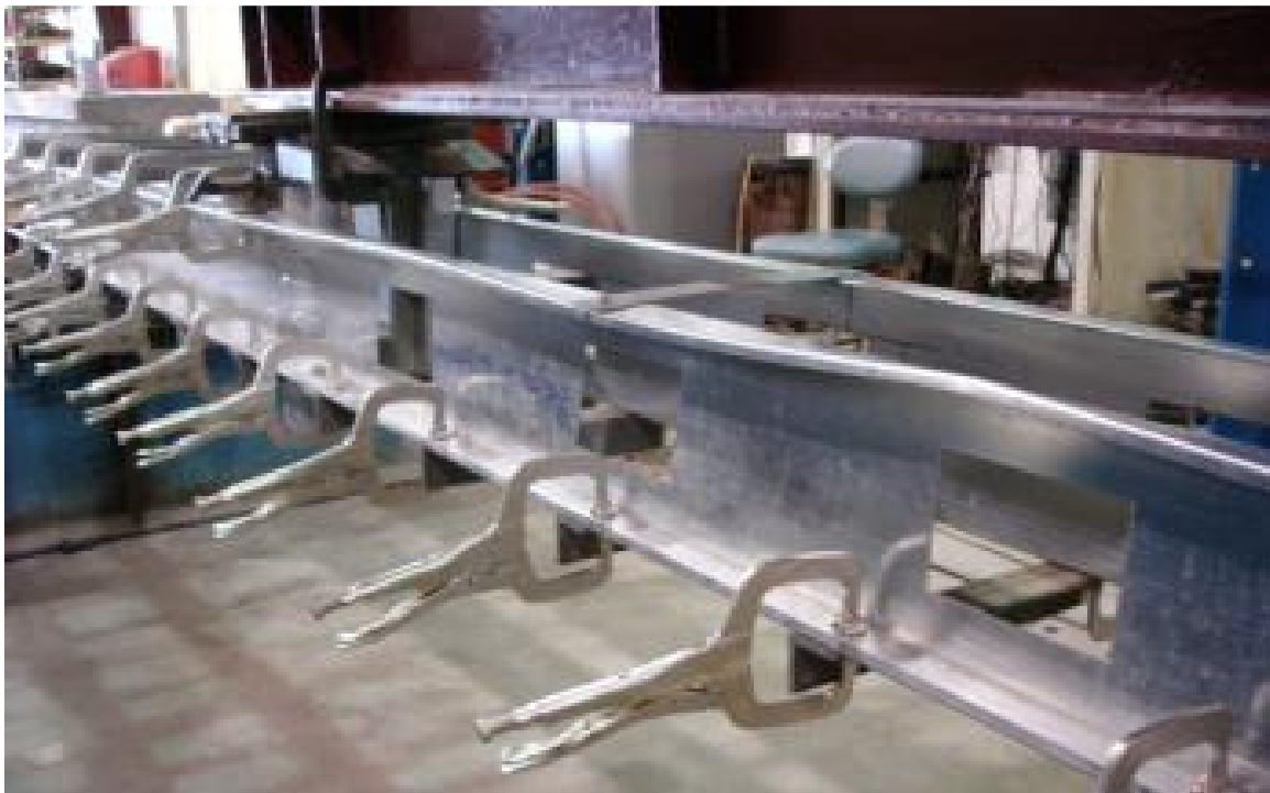
Figure 4.2. Distortional buckling of the compression flange (beam 800S200-33-95-3-2)
