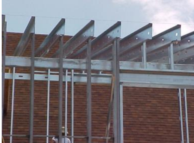
Figure 1.3. Web holes are provided in the roof purlins (photo courtesy of Steel framing)
