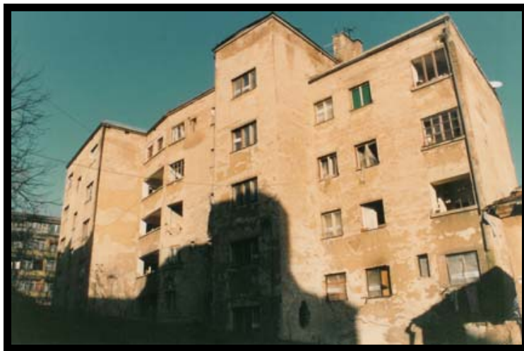
Figure 3.2. Building in the midst of war (1993). Picture of the Alipašina 7 building (the rear view). During the course of the war the building sustained over 13 direct hits (photograph courtesy of Amra Kurtagic, 1993).
