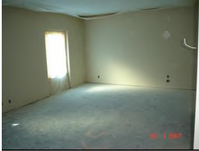
Figure 2.2 Hampton Inn Building at the Time of Testing
