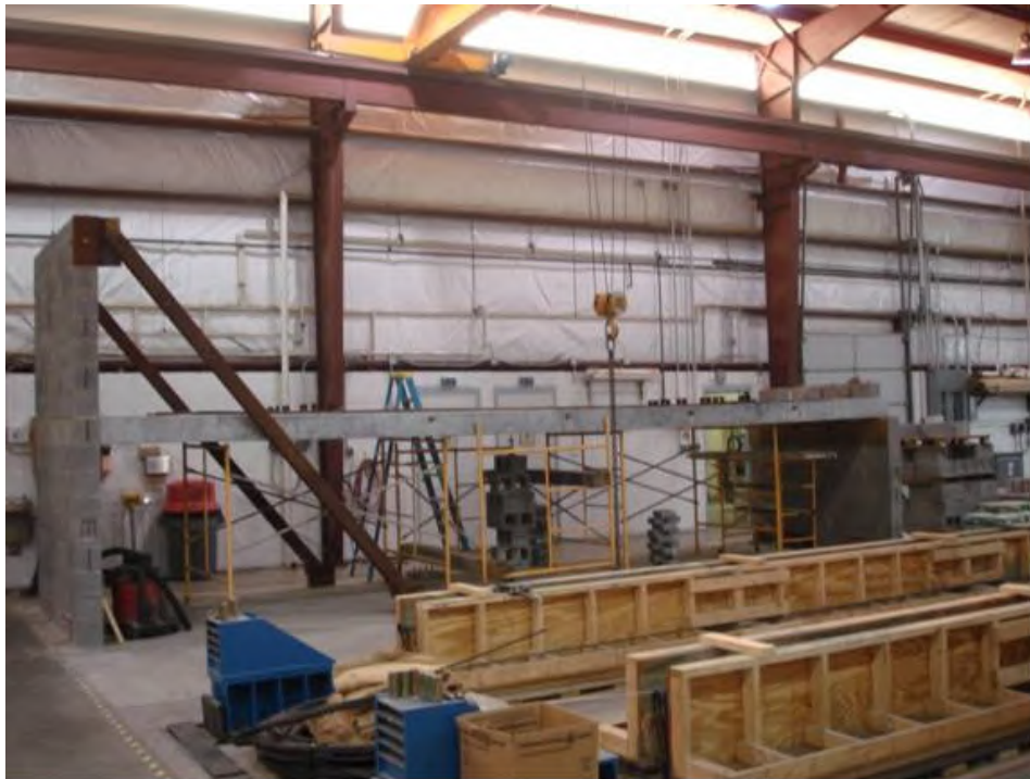
Figure 3.8 Left Upper Wall with Braces (Stage 2)
