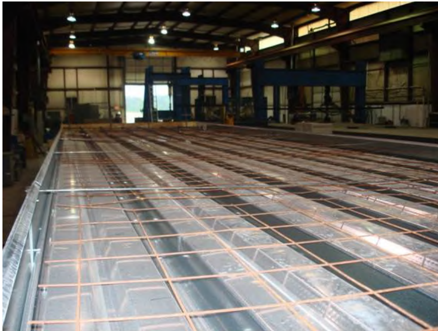
Figure 3.6 Cold Formed Steel and Plywood Pour Stops
