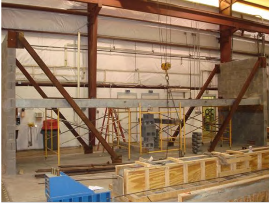
Figure 3.9 Right Upper Wall with Braces (Stage 3)
