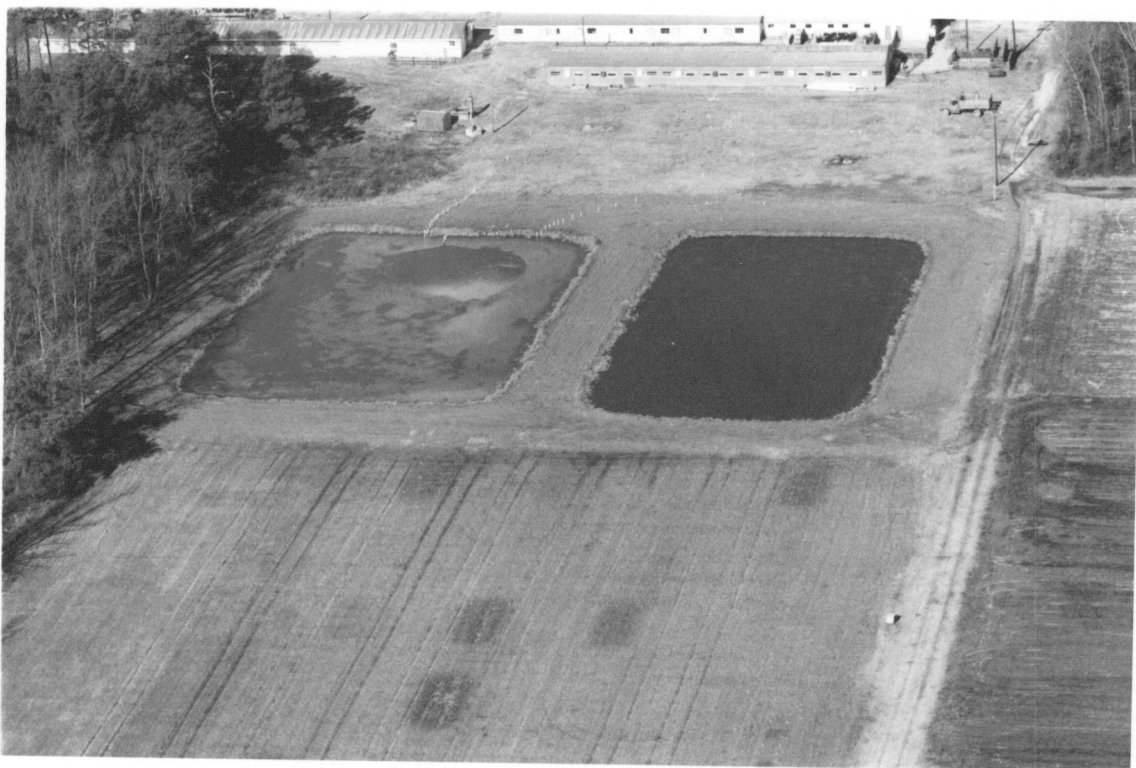
Fig. 1 Holland Station anaerobic lagoon on left and aerobic lagoon on right. Two series of wells are visible at top center of photograph.
