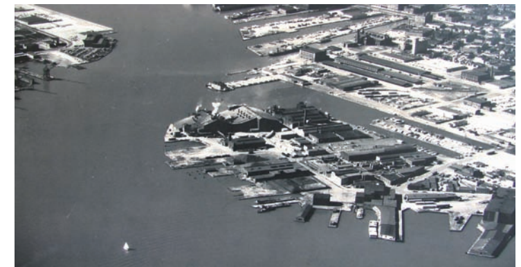
Bird's eye view of the site and the textile factory
