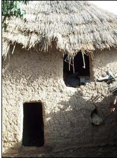
Figure 3-3. Storage of pesticides in an unsecure room.
