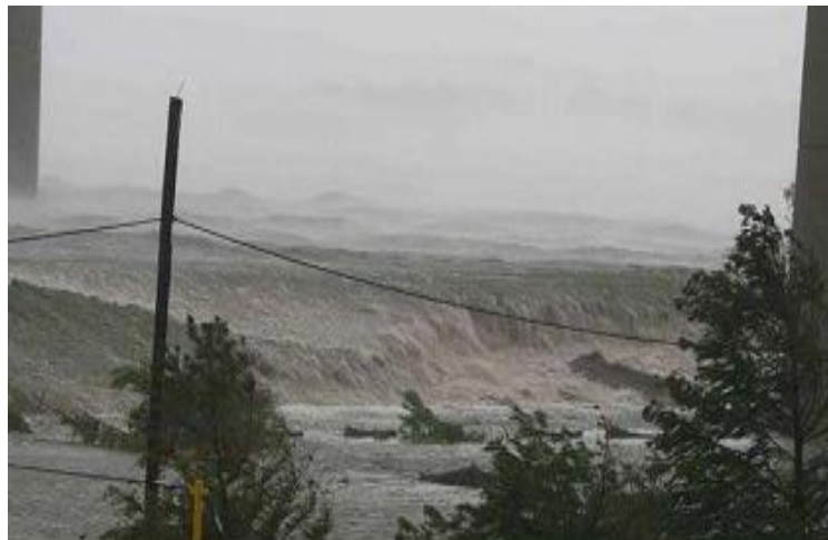
Figure 3 - Levee Overtopped During Hurricane Katrina (Murdock, 2007)
