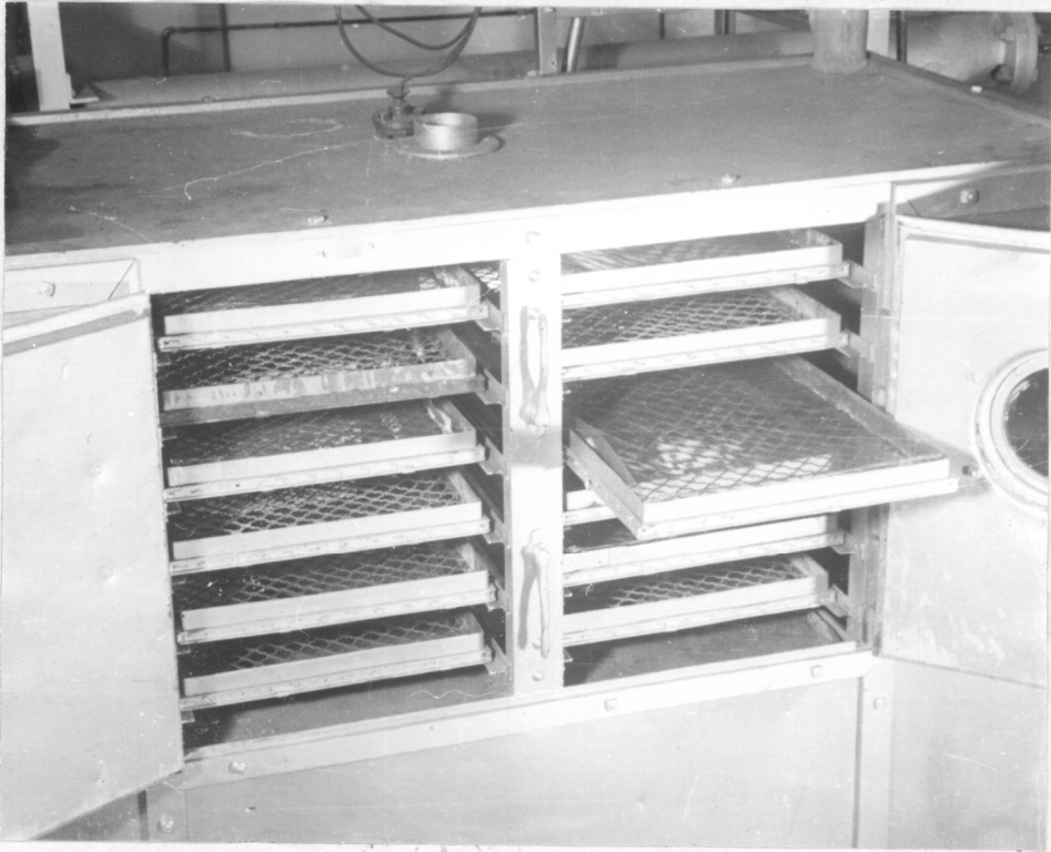
Proctor and Schwartz Atmospheric Tray Drier
