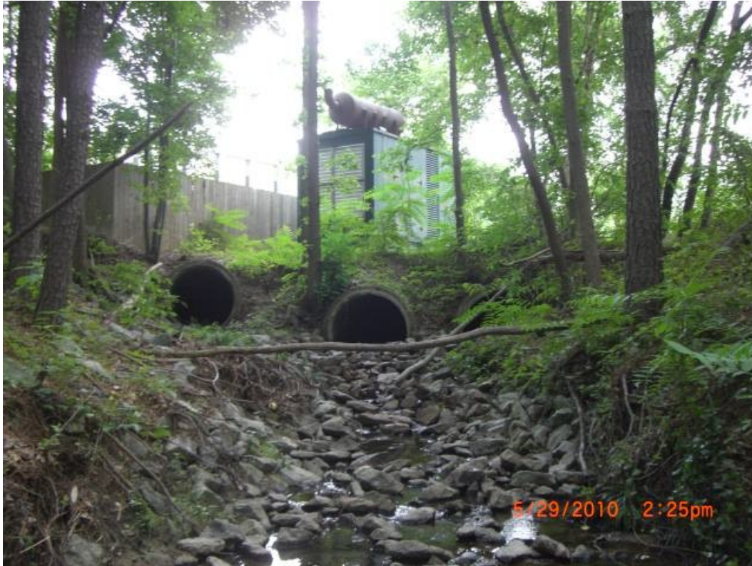
Figure 30. Culverts from parking lot in P19 watershed. Photo by author, 2010.
