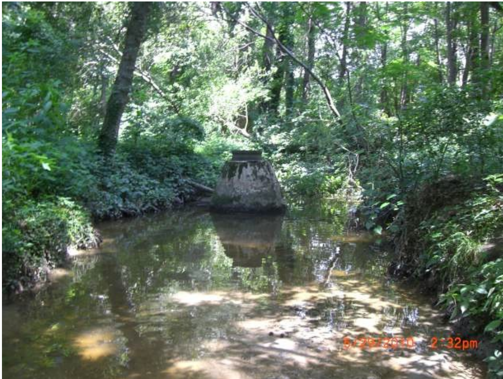
Figure 31. Example of one of the two sewer manholes interfering with the stream in P19. Photo by author, 2010.
