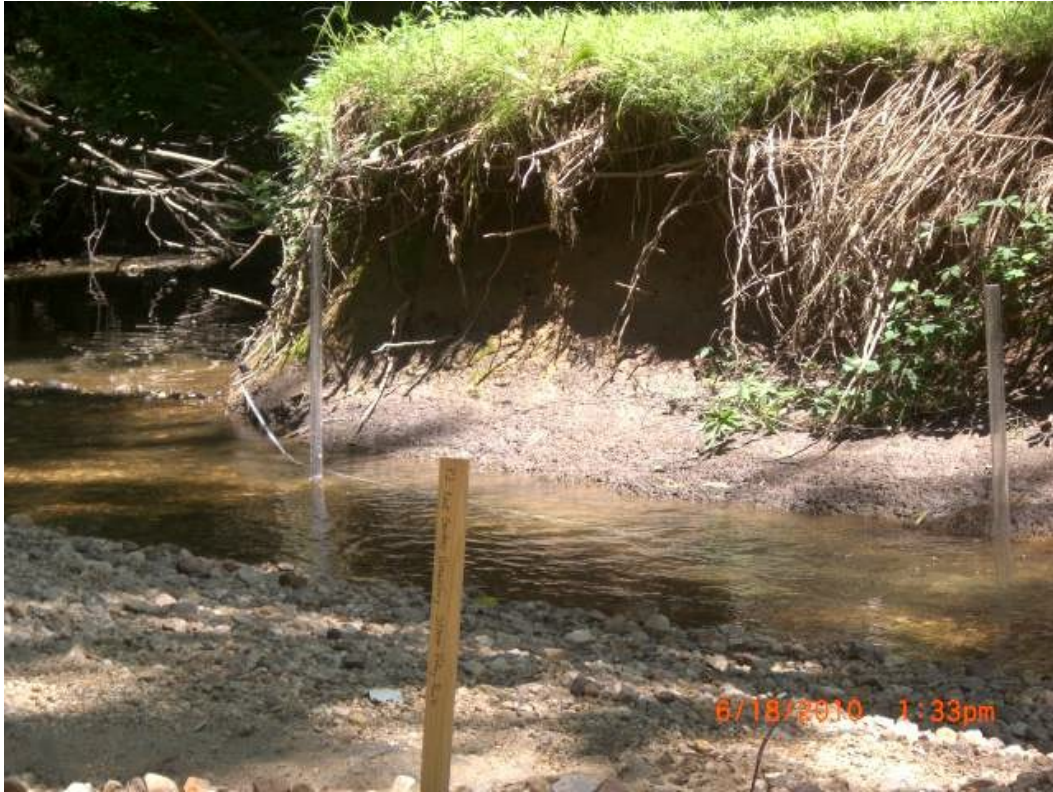
Figure 8. Eroding stream bank exposing clay layer at field site P2. Photo by author, 2010.
