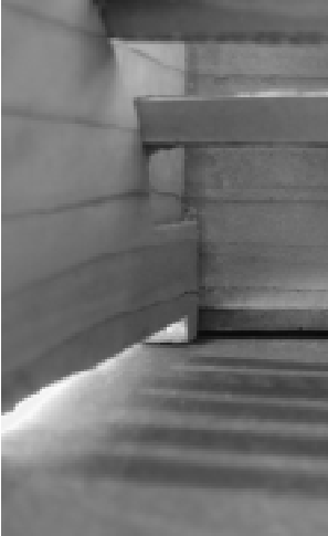
plastered concrete beams with a spherical exterior section, conical interior section
