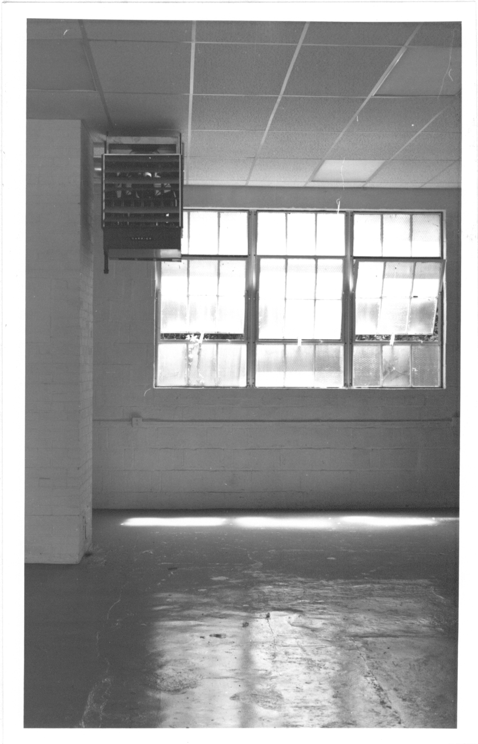
Figure 3. PHOTOGRAPH OF WORK AREA
