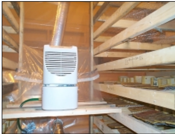
Figure 3.17: Dehumidifier positioned inside the climate chamber.
