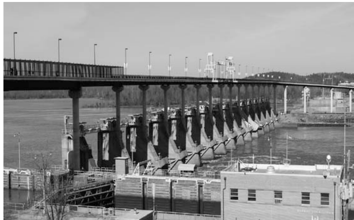
Fig 1. Murray lock and dam, Arkansas River
