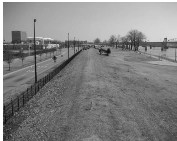
Fig 7. Levee along NLR riverfront
