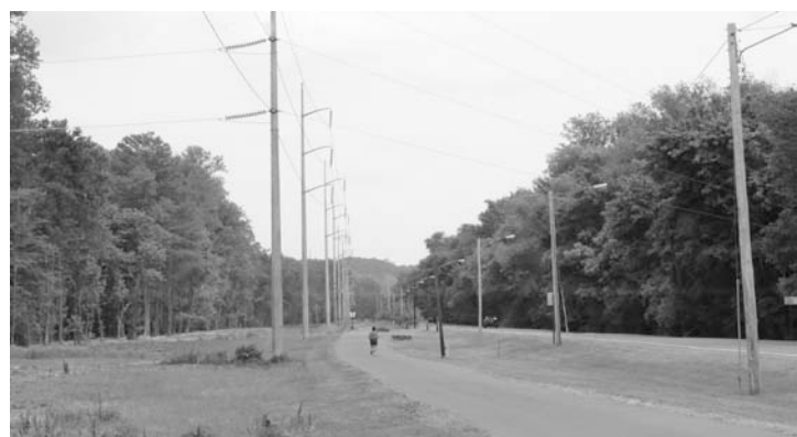
fig 3. linear power line easements
