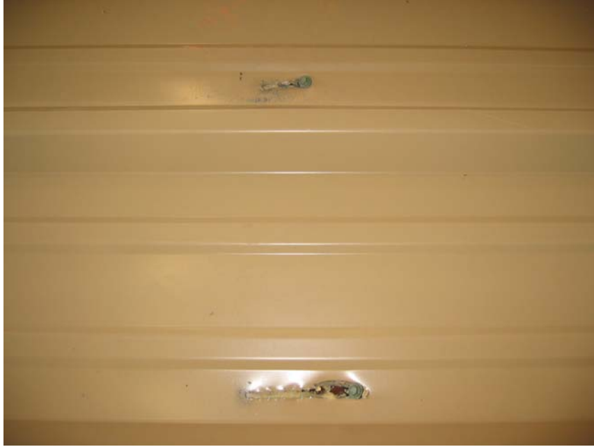
Figure 3.10. Bearing Failure in Deck
