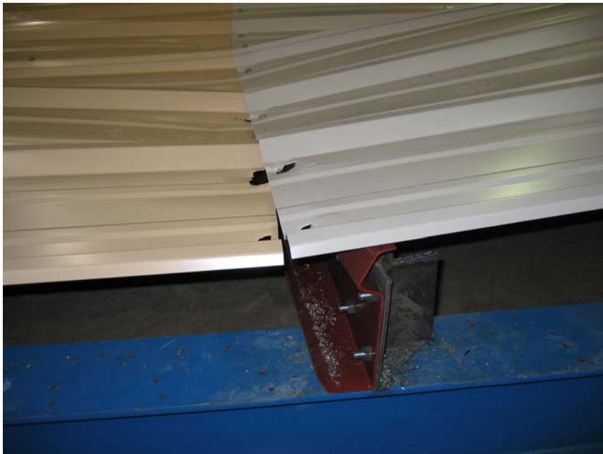
Figure 3.11. Bearing Failure in Deck
