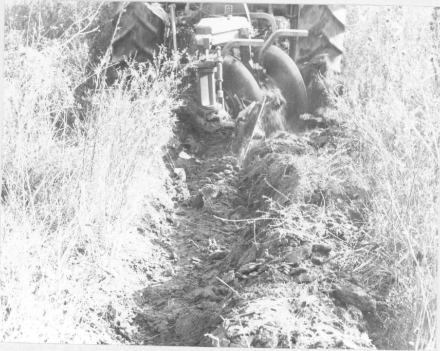
Figure 4. Plowing furrow for the erection of the portable fence.
