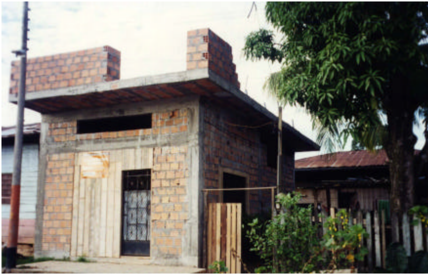
Photo A.6. A house constructed with the assessment and support of the Ministerio de Construcción y Vivienda
